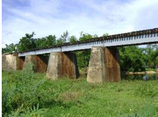
Note: This bridge is listed in the 132 bridges group. Source: TRICC [Fig. 3-1-24] Bridge at 812k168m <No.6/132>
