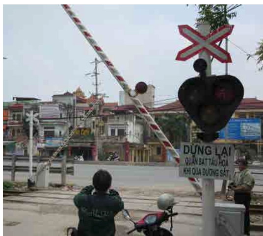
(a) Warning signal and barriers during automatic operation
