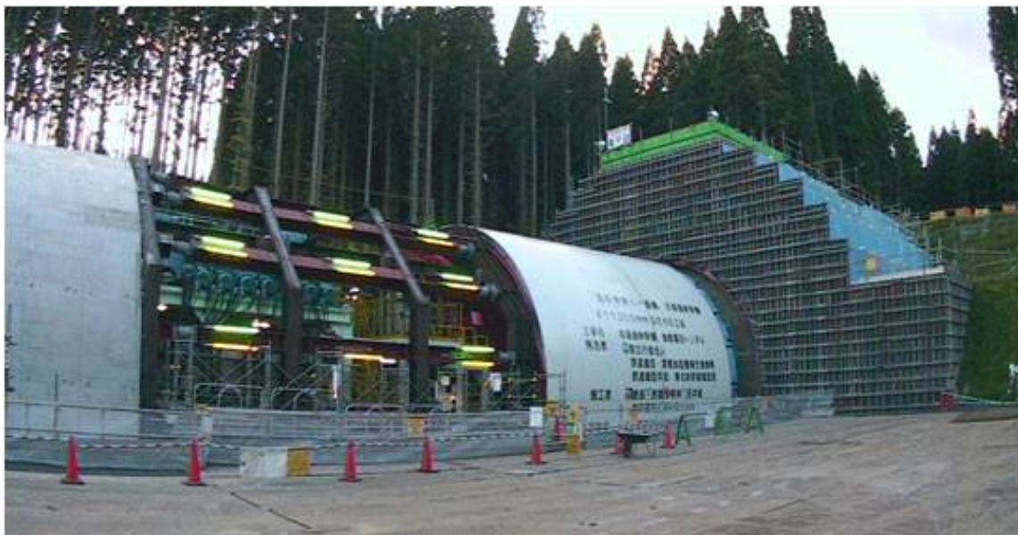
[Fig. 8-4-7] Improved SENS Shield Machine
