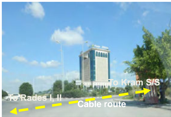
Figure 7.2.3-14 Cable Route (Point A)
