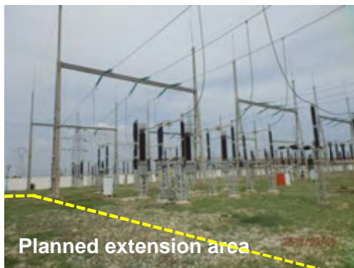
Figure 7.2.3-7 Existing Mnihla S/S
