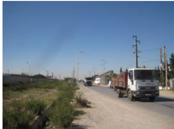
A 7 m wide, two lanes road from the crossing to the prospective carry-in entrance of the site. The distance between light poles and electric poles is 14 m.
