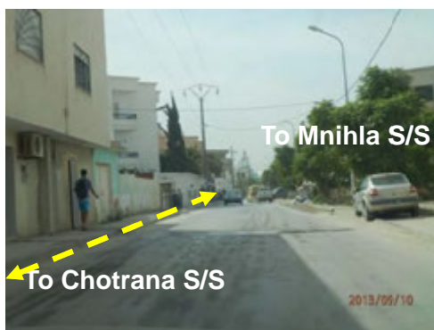
Figure 7.2.3-20 Cable Route (Point A)
