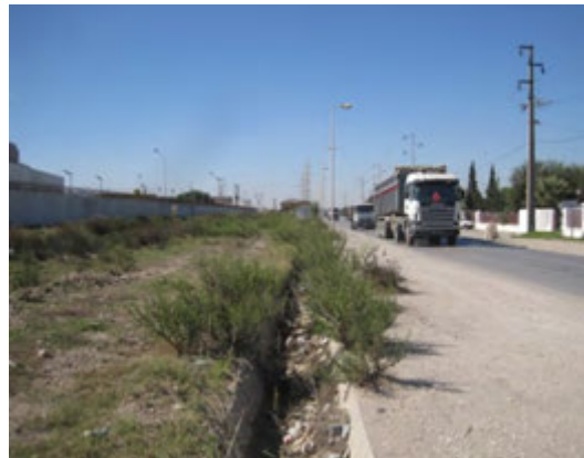
There is a small drain of 1 m width and 0.7 m depth along the road.
