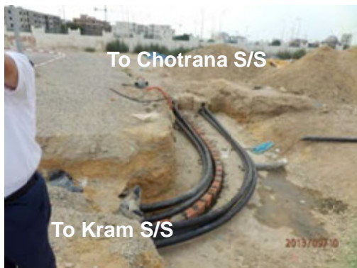
Figure 7.2.3-17 Cable Installation (Point A)
