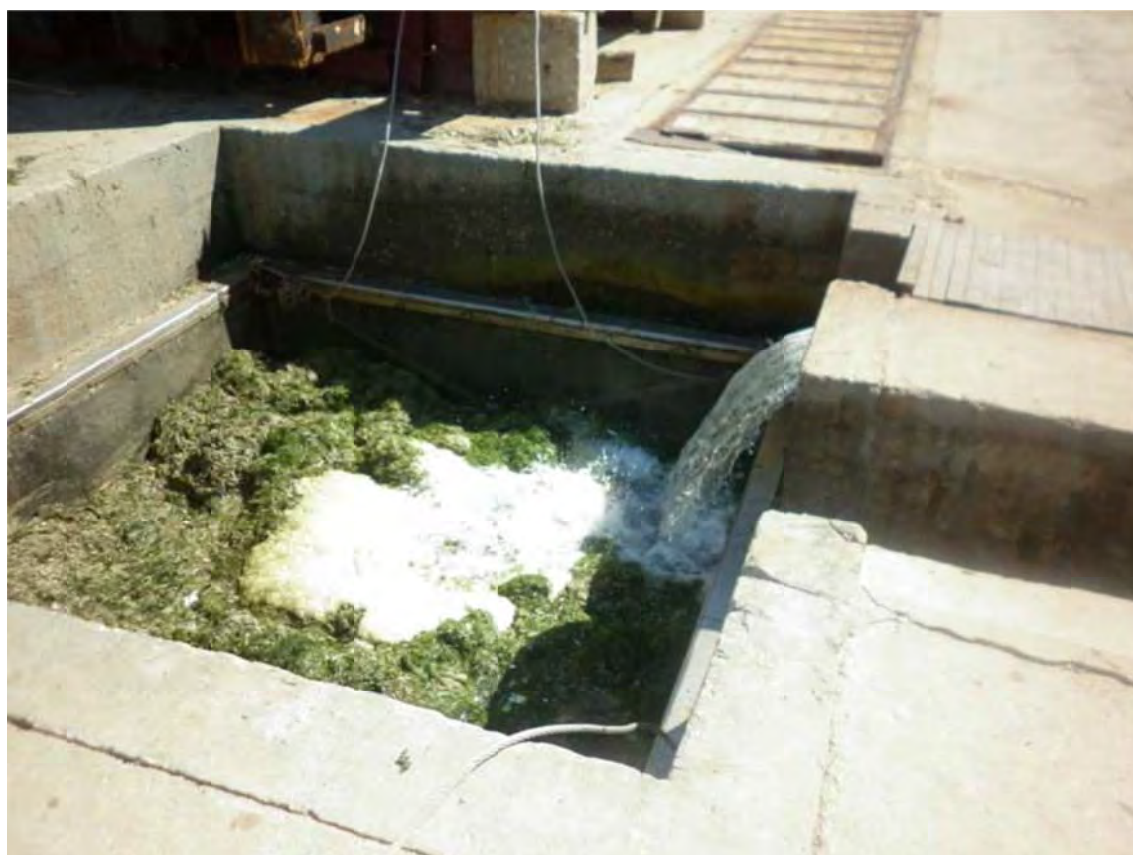
Figure 8.7-14 Sediment, Sea-grass etc.. Retained in the Gates of the Pumping Station
