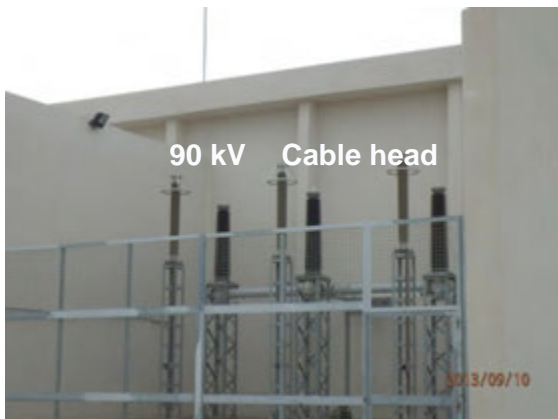
Figure 7.2.3-1 90 kV Cable Head of Kram S/S
