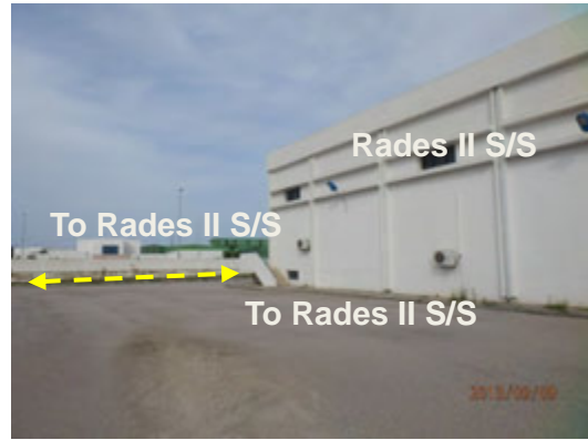
Figure 7.2.2-8 Planned are for installing Cablese near Rades II S/S (PointB)
