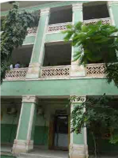
▲ School building of ATI
