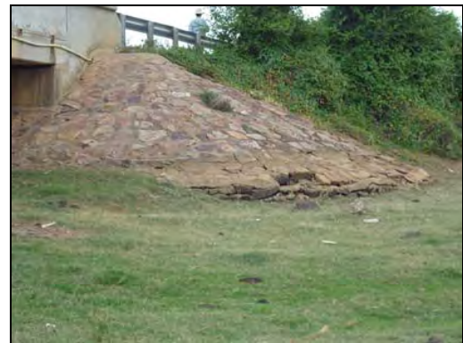
Br. 60 View on Pursat Side Abutment
