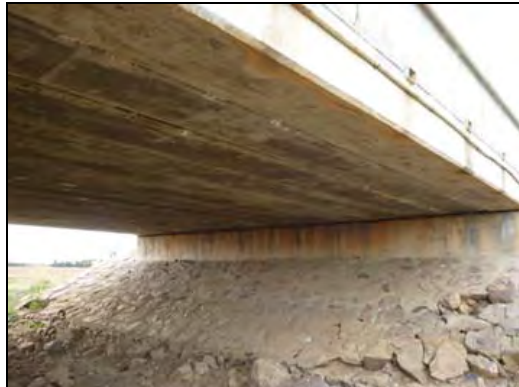
Br. 61 View on Phnom Penh Side Abutment
