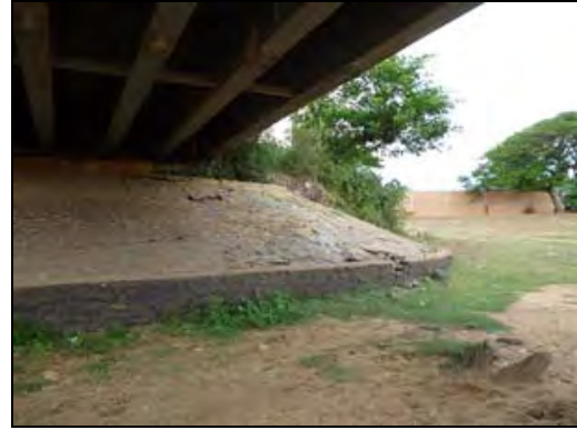
Br. 59 View on Phnom Penh Side Abutment
