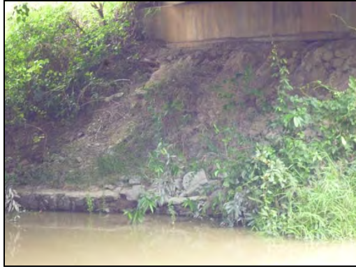
Br. 40 View on Pursat Side Abutment
