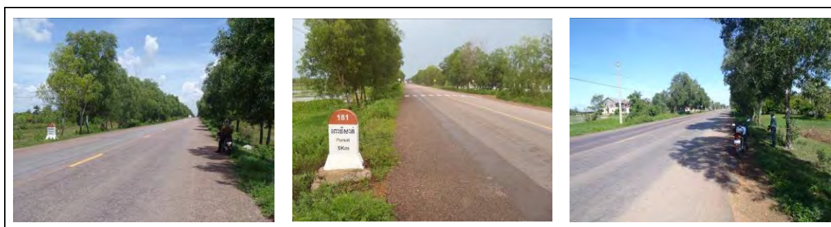
Figure 15.2-9 Roadside Trees along NR 5
