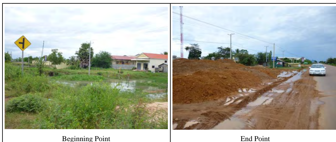
Figure 8.4-3 Photo at Pursat Bypass Route
