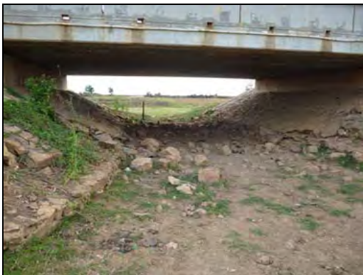
Br. 61 View on Abutment
