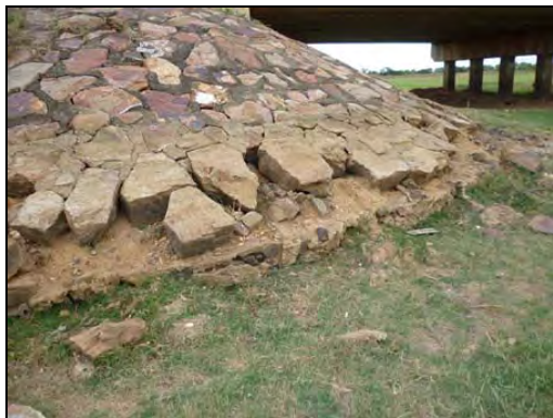
Br. 60 View on Phnom Penh Side Abutment
