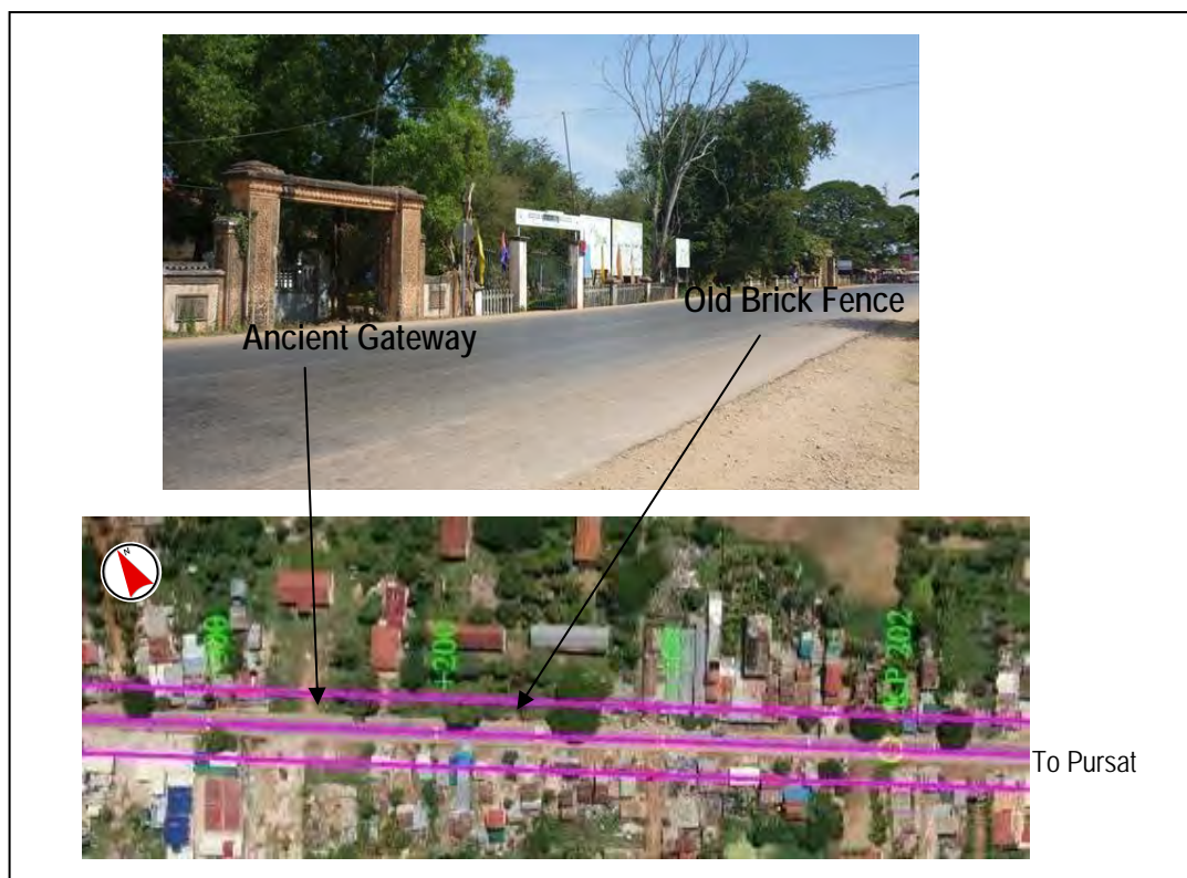
Figure 15.3-11 Brick Fence and Gateway of Royal Palace of Preah Bat Monivong
