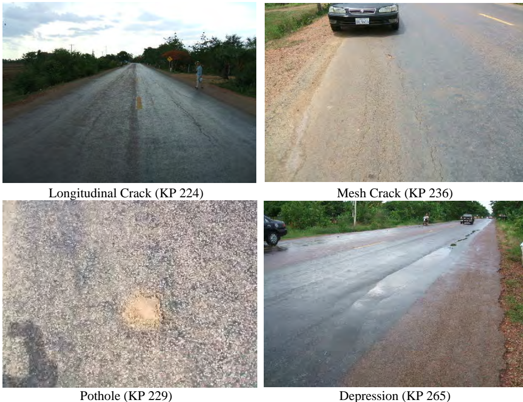
Figure 4.1-1 Condition of Middle Section
