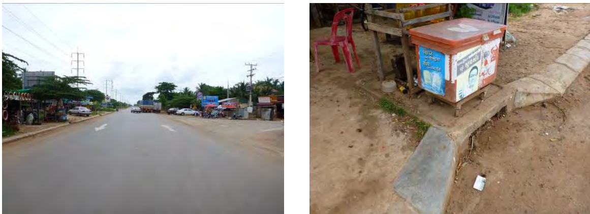
Figure 4.2-6 Road Surface Lower than Adjacent Land in the Commercial Area (Left) and Inlet of Drainage Installed under CRIP
