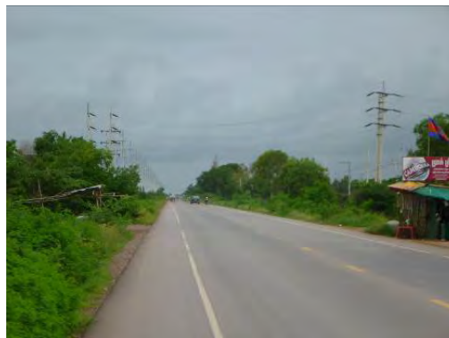
Figure 4.6-8 Electric Power Line in the Vicinity of KP 186
