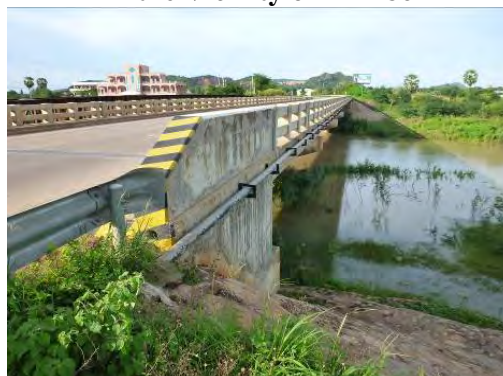
Figure 4.6-9 Telecommunication Cable at KP 365 + 800
