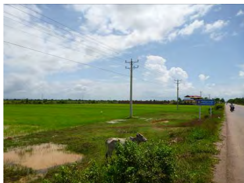
Figure 4.6-1 Electric Poles near KP 214
