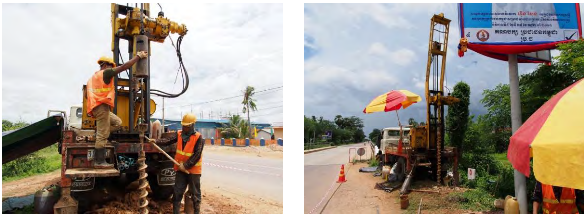
Figure 6.4-4 Truck-Mounted Rotary Auger, with SPT Apparatus
