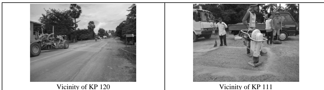
Figure 3.4-2 Pavement Repair by RAMP Project
