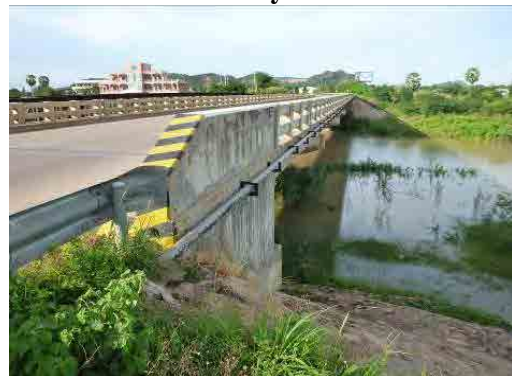
Figure 4.6-9 Telecommunication Cable at KP 365 + 800
