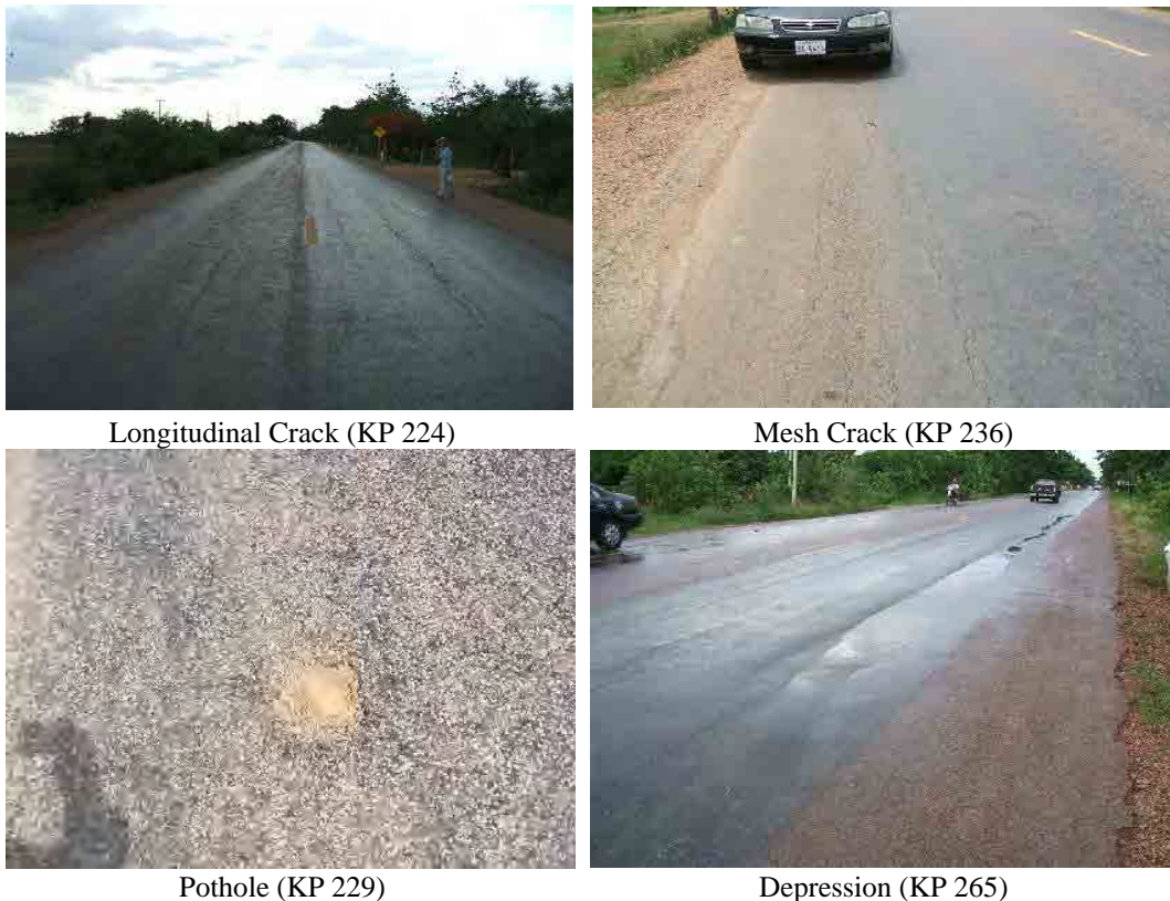
Figure 4.1-1 Condition of Middle Section
