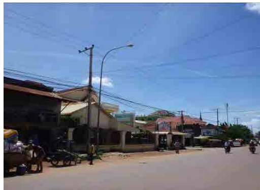
Figure 4.6-5 Street Light near KP 367
