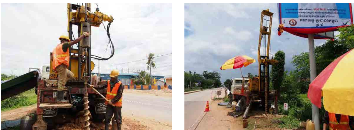
Figure 6.4-4 Truck-Mounted Rotary Auger, with SPT Apparatus
