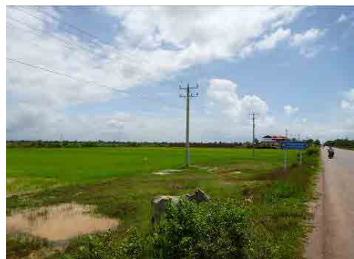
Figure 4.6-1 Electric Poles near KP 214
