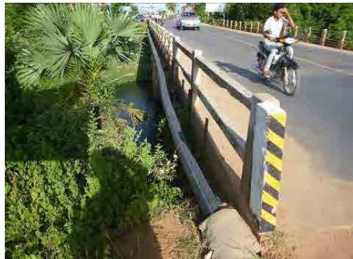
Figure 4.6-3 Water Supply Pipes on Br. 48 (KP 187 + 500)
