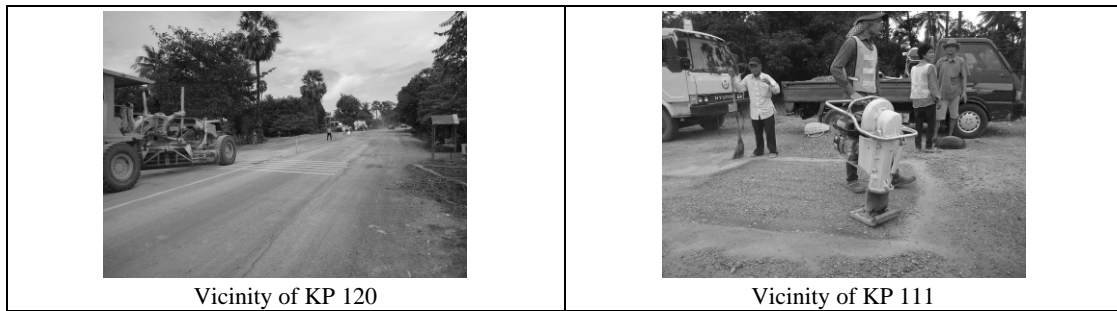
Figure 3.4-2 Pavement Repair by RAMP Project
