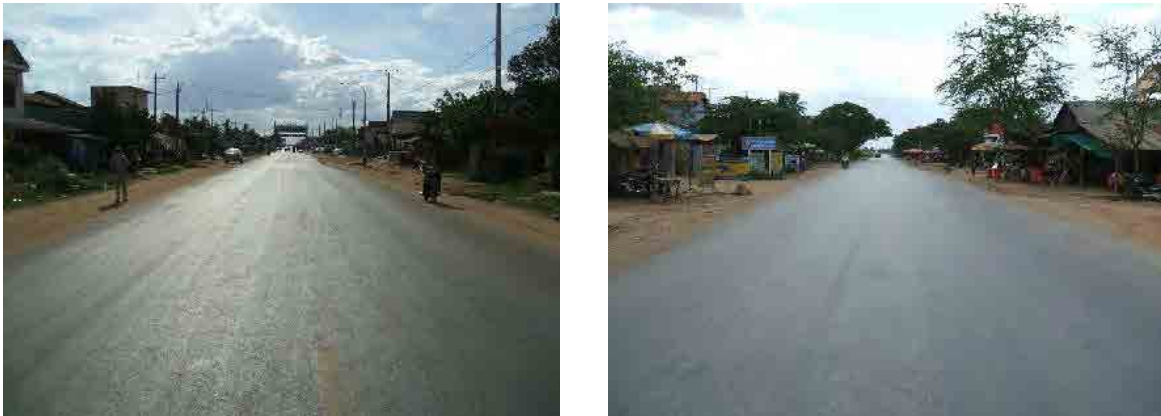
Figure 4.2-3 Road Surface Lower than Adjacent Land; Inundation Occurred due to Rain Water Flowing into Road from Adjacent Land
