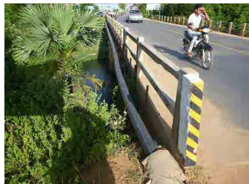
Water Supply Pipe at Br. 48 (KP 187 + 500)
