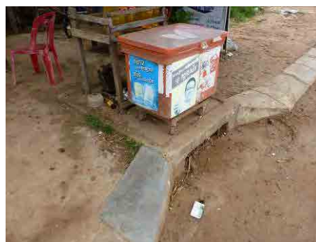
Figure 4-6 Inlet of Drainage
