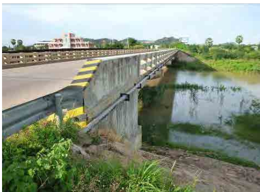
Telecommunication Cable at KP 365 + 800
