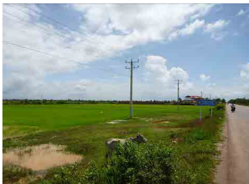
Electric Pole in the Vicinity of KP 214
