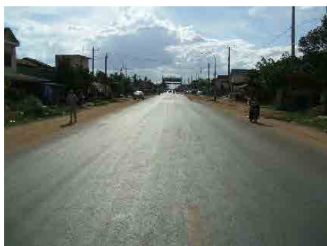
Figure 4-5 Road Lower than Adjacent Land
