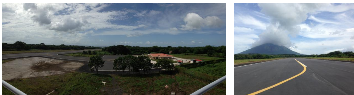
Figure 20.10.1 Airport Facilities and Runway views from Ometepe Airport
