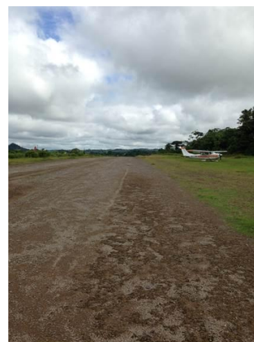
Figure 20.5.1 San Carlos Airport Runway View
