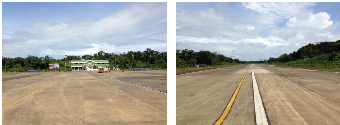
Figure 20.9.1 Airport Facilities and Runway views from San Juan de Nicaragua Airport
