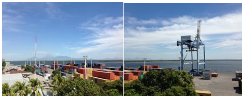
Figure 8.4.4 Container Yard and Gantry Crane at the Puerto Corinto Port
