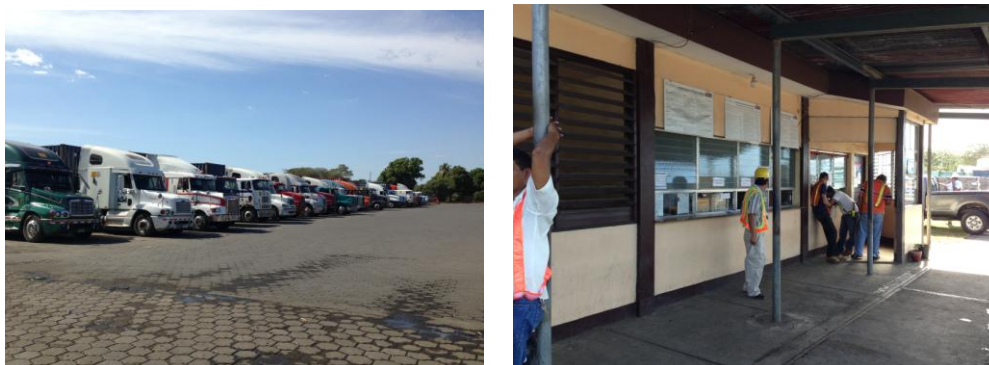
Figure 8.4.5 Truck Terminal and Customs Office
