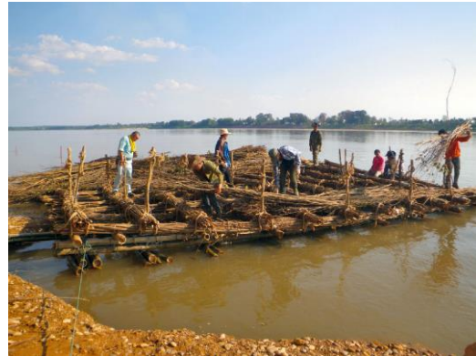
Photo 3.4-18 Installation Method of Soda Mattress in Previous Pilot Construction (Left: IDI Pilot Construction (2001) and Right: Pakthoay Site in Bolikhamxay Province (2013))
