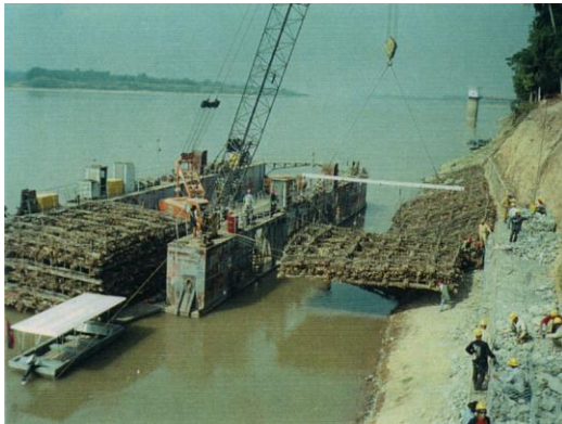
Photo 3.4-18 Installation Method of Soda Mattress in Previous Pilot Construction (Left: IDI Pilot Construction (2001) and Right: Pakthoay Site in Bolikhamxay Province (2013))
