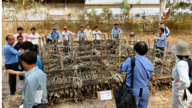
Photo 3.3-6 Completed 4m × 4m Soda Mattress (Minimum Size)
