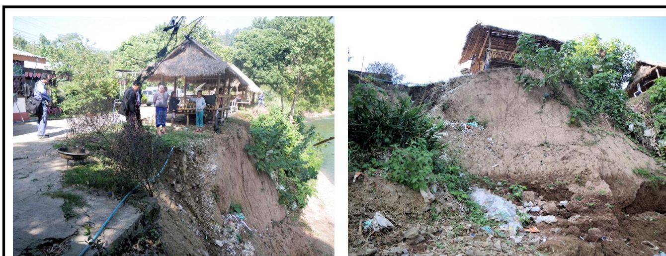
Before Construction (December 2010)
