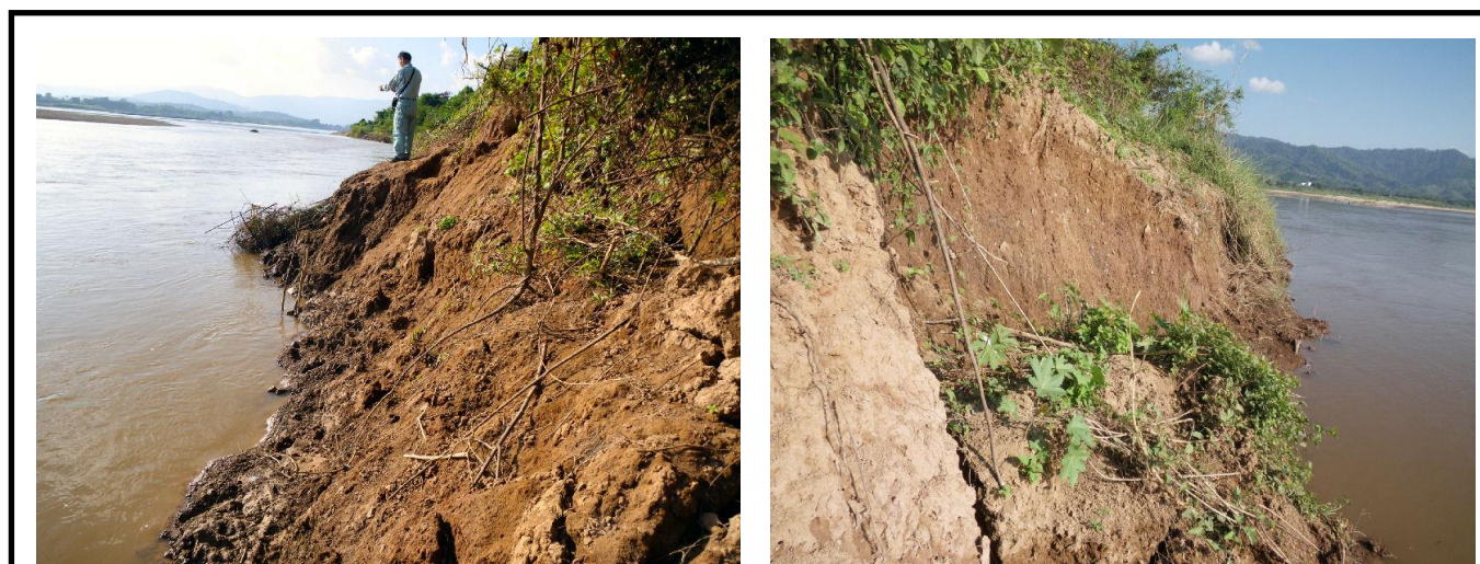
Before Construction (December 2010)
