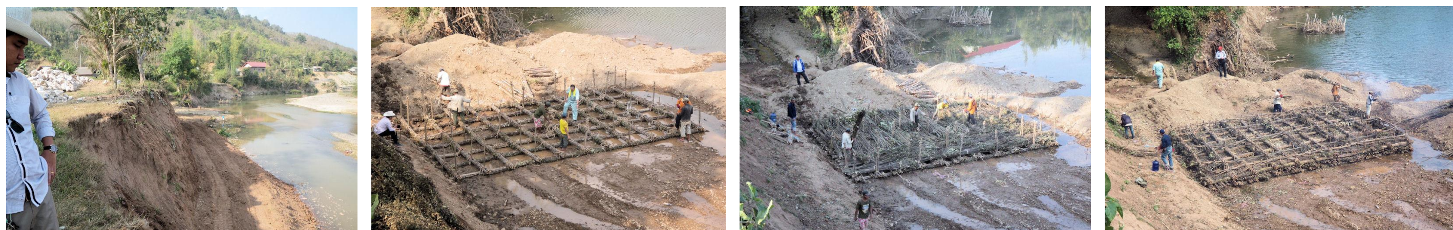
During Construction (February 2014)
