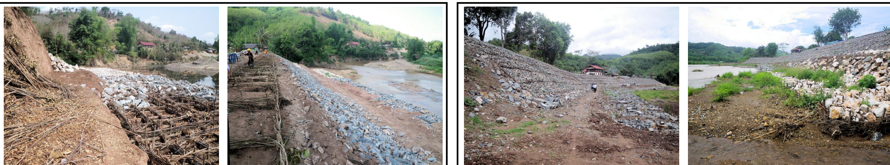
During Construction (From March 2014 to May 2014)
