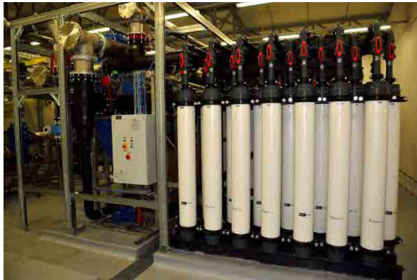
Installed Water Treatment Facilities (UF Membrane and Back Wash Pump)
