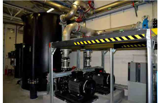
Installed Water Treatment Facilities (UF Membrane and Back Wash Pump)
