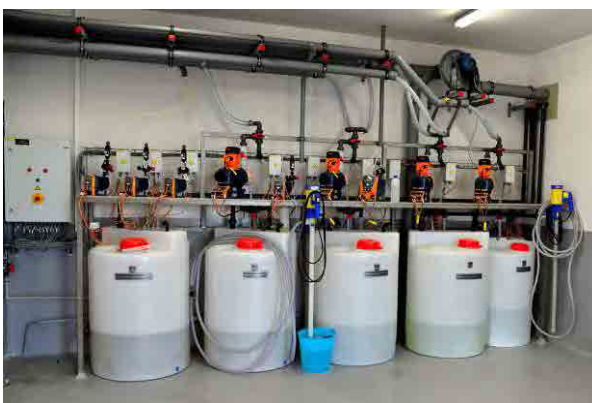
Installed Water Treatment Facilities (Chemical Dosage Equipment and Neutralization Tank Equipment)
