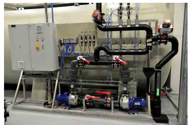
Installed Water Treatment Facilities (Chemical Dosage Equipment and Neutralization Tank Equipment)
