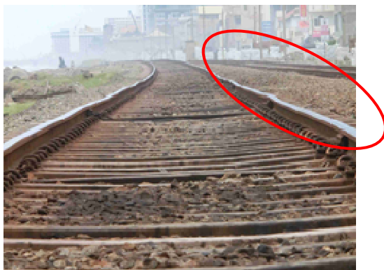
Figure 1.6.5 Irregularity of Alignment
