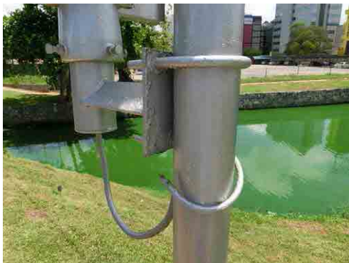
Figure 1.6.17 Exposed Terminal Box
