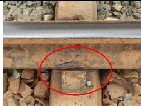
Figure 1.6.8 Snapped Fastener
