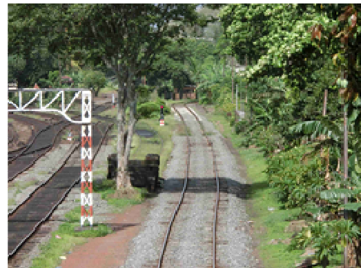
Figure 1.6.6 Irregularity of Alignment
