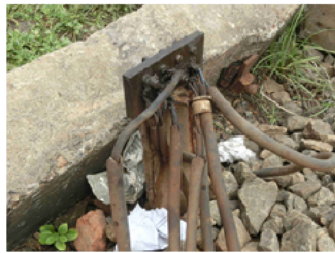
Figure 1.6.18 Broken Fastener
