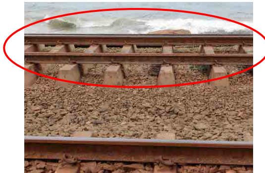
Figure 1.6.9 Exposed Sleepers
