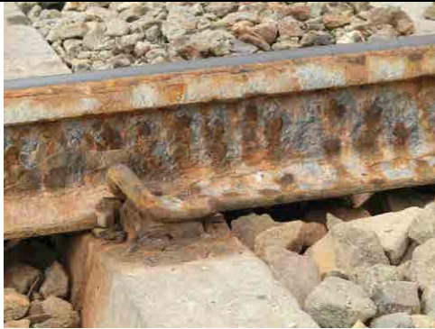
Figure 1.6.7 Corroded Rail
