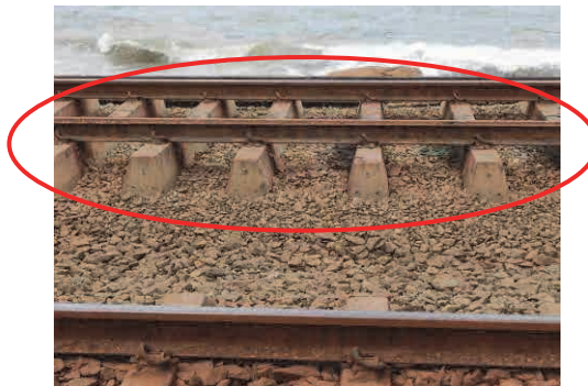
Figure 3.2.13 Exposed Sleepers
