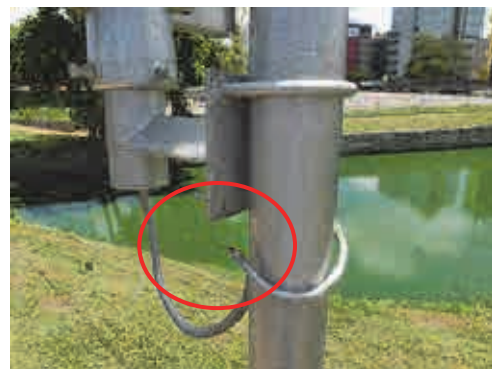
Figure 3.2.15 Exposed Terminal Box
