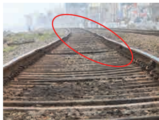
Figure 3.2.12 Irregularity of Alignment
