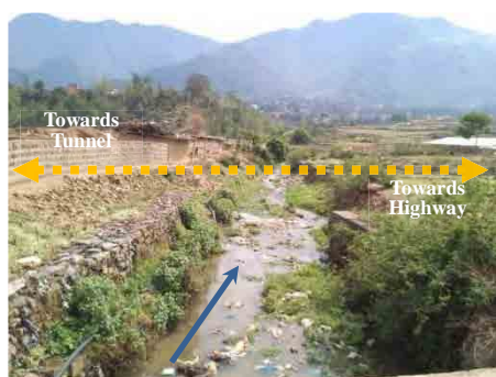
(a) Proposed Culvert Site
