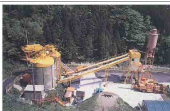
(b) Shotcrete Mixing Plant
