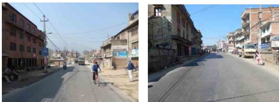
Photos 4-3 Insufficient (Unsecured) Right-of-Way at Built-up Areas
