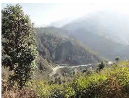
Jhyaple khola Collapse
