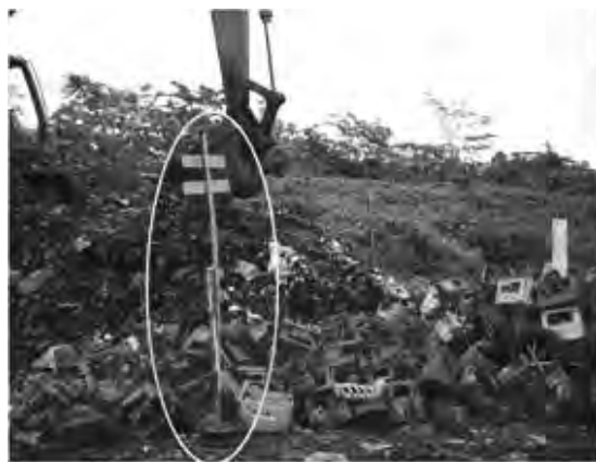
Photo 3-12: Height control with a wooden post
