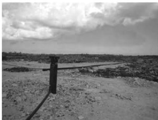
Soil coverage around the wells to extract methane gas in the CDM project (May, 2011)
