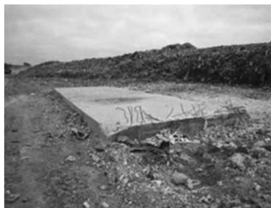
Photo 3-17: Basement for truck scale, 8 vías
