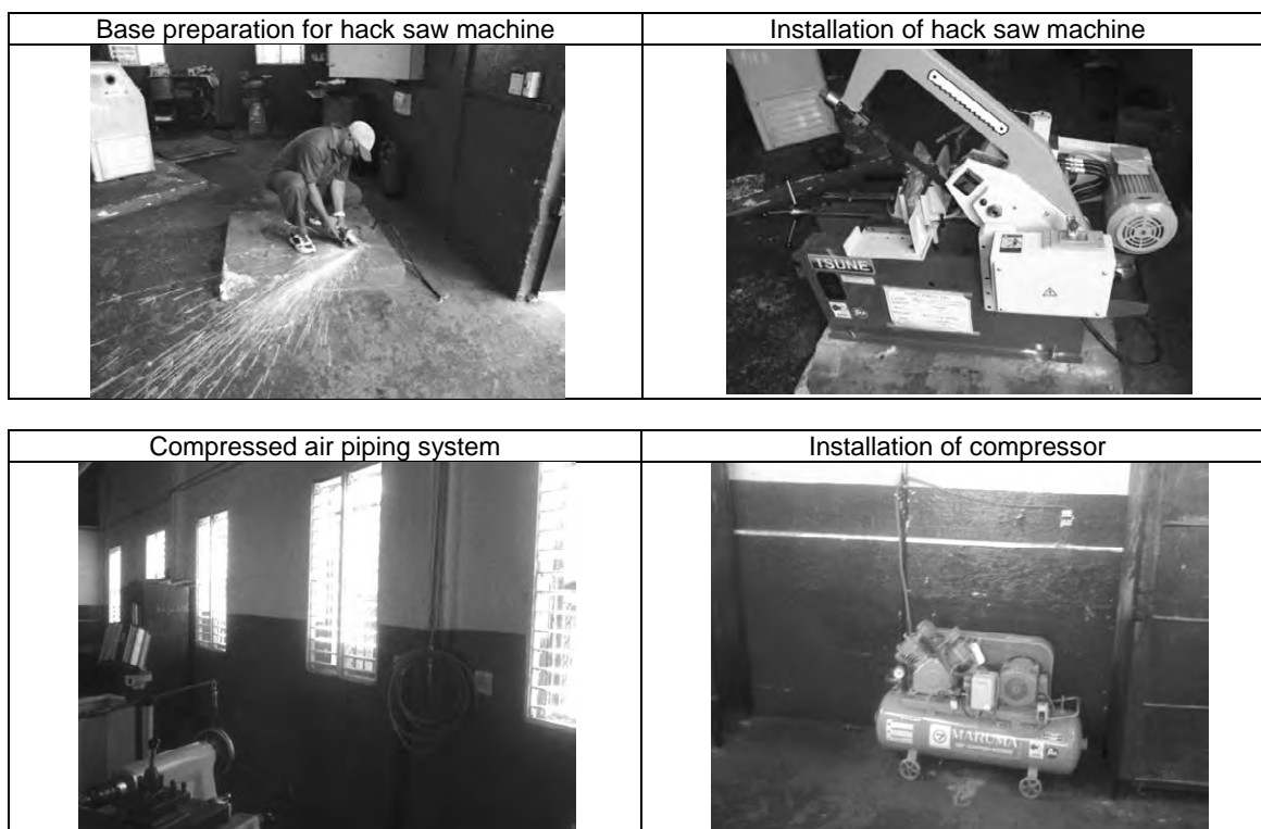
Photo 7-2: Machine Workshop (Hack Saw and Air Piping System)
