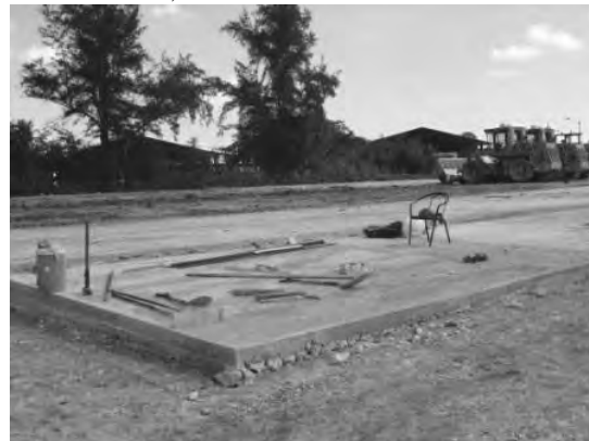
Paving of parking area for heavy equipment: paved area 65m x 73m = 4,745 m 2
