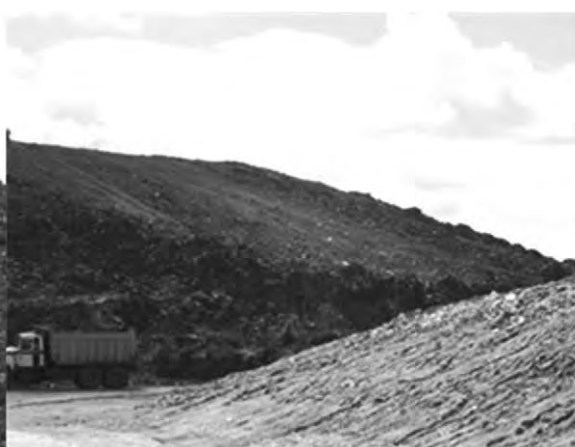
Photo 7-4: Site condition after the fire was quenched and the wastes were covered with soil
