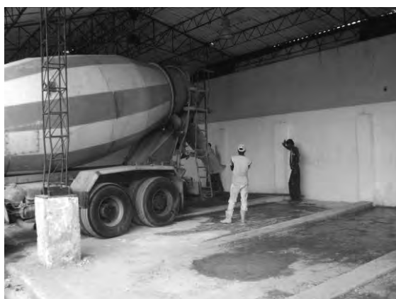
Photo 1-5: Pouring concrete for the plant floor (February 13, 2012)
