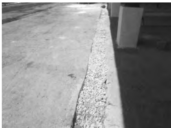
Photo 1-24: Drainage using gravel
