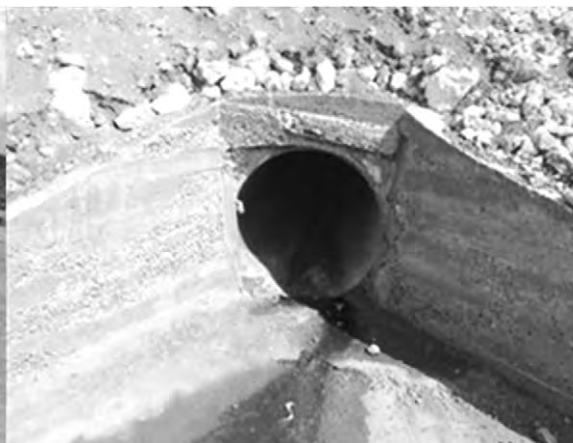
Photo 7-8: Crossing pipe construction
