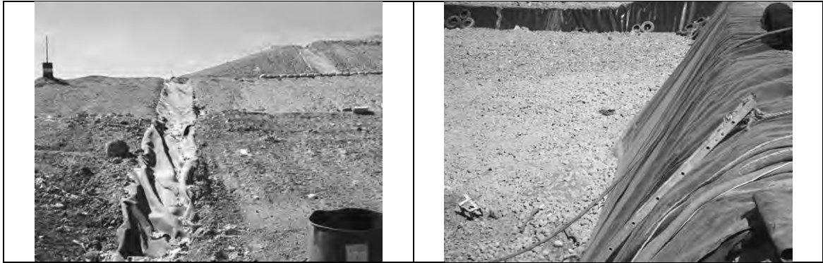
Photo 1-3: Surface drainage and Impermeable Liner
