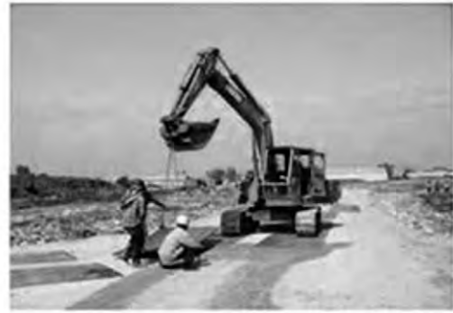
Construction of Main Road
