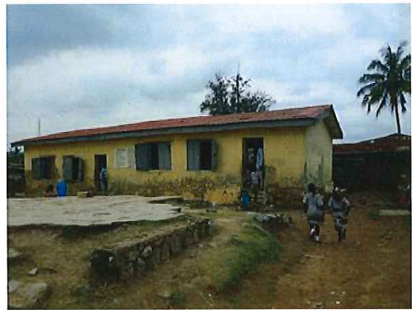
N1-P1 RATIBI MOSLEM PS ODINJO (Congested and deteriorated facility)
