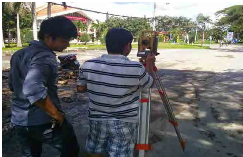
Photo 1: Positioning boreholes in the field
