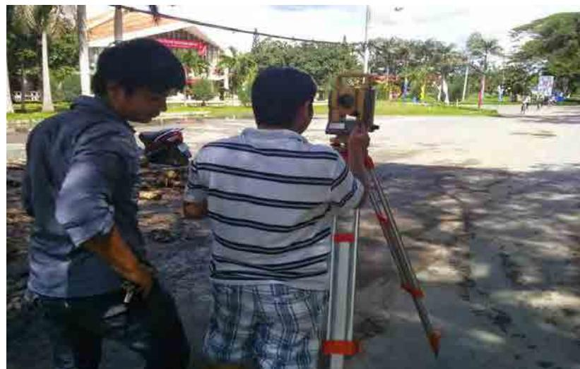
**Photo 1: Positioning boreholes in the field**
