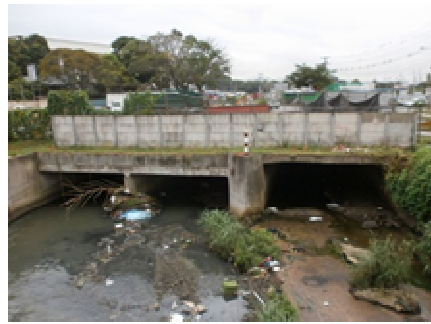
Photo 2: River Box-Culvert
