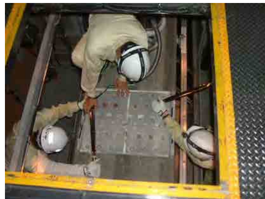
Inspection of Track Bolts [ Okinawa Urban Monorail ]
