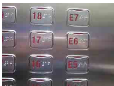
Braille indications for blind people in elevators
