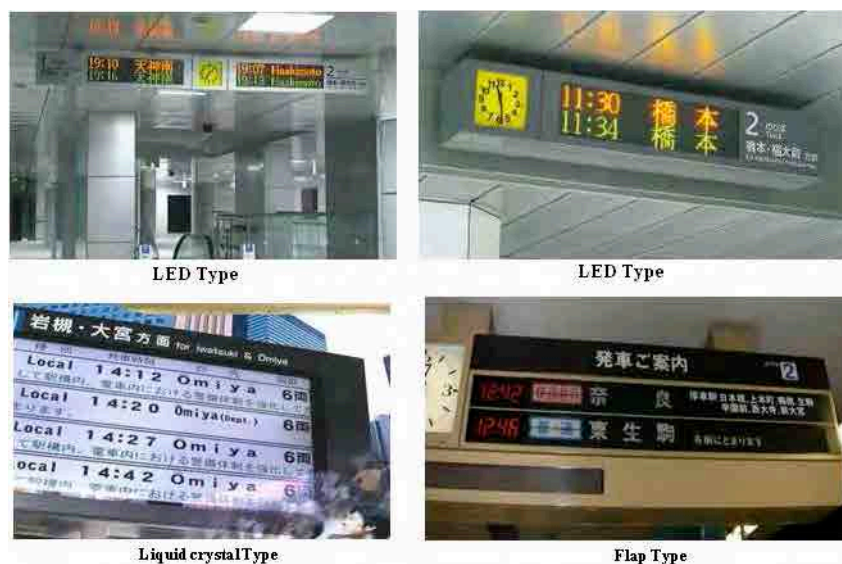
Source: JICA Study Team Figure 7.65 Example of Passenger Information Display Systems (PIDS)
