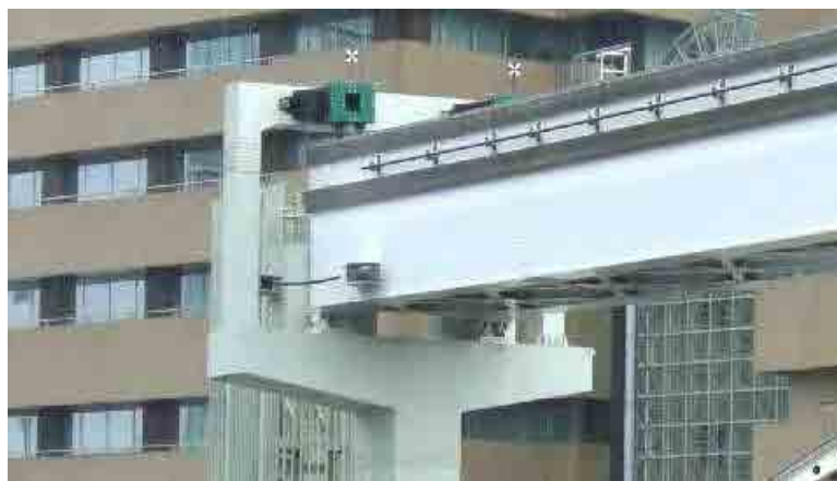
Figure 7.18 Photo of the stoppers, (Sample: end of Tama Monorail)
