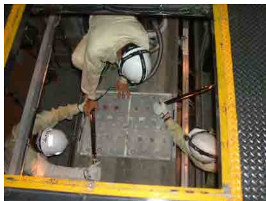
Inspection of Track Bolts [ Okinawa Urban Monorail ]
