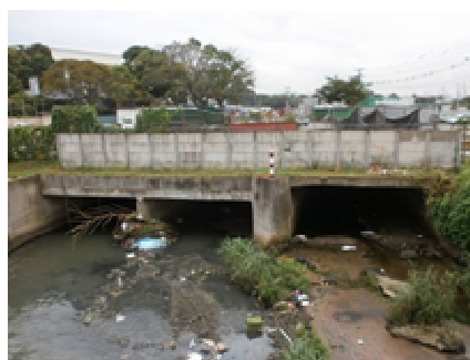
Photo 2: River Box-Culvert
