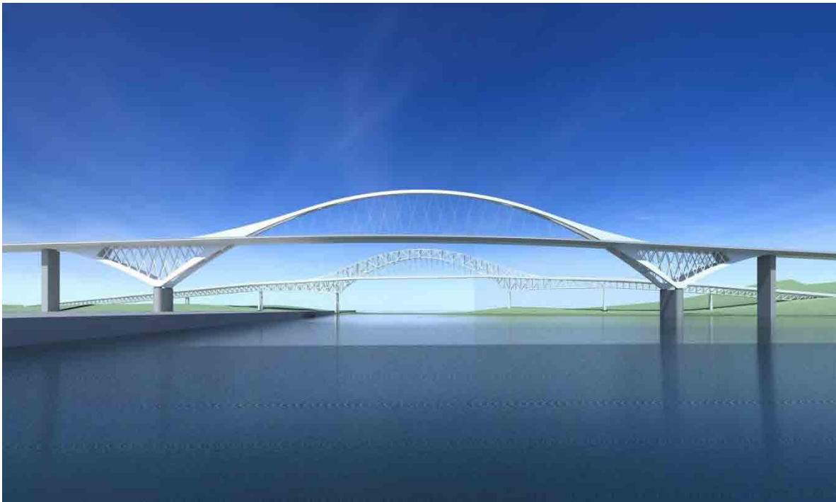
Figure # 2 Steel Arch Bridge Type
