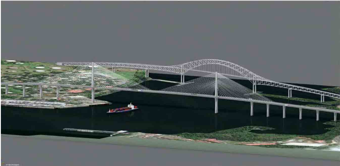
Figure # 1 Cable-Stayed Bridge Type
