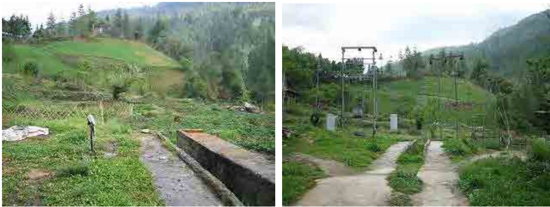
Figure 5-2 Training area of CMTD Begana (left: May 2012 right: May 2014)
