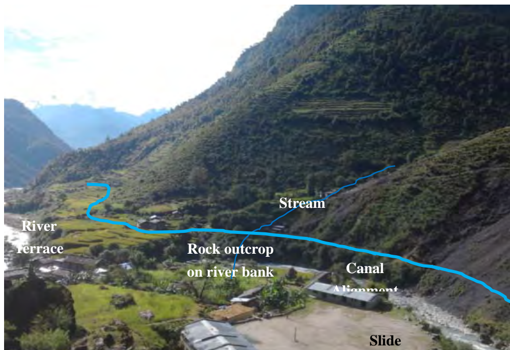
Figure 7-10 Middle Part of the Canal Alignment (Photograph taken from the Opposite Bank)
