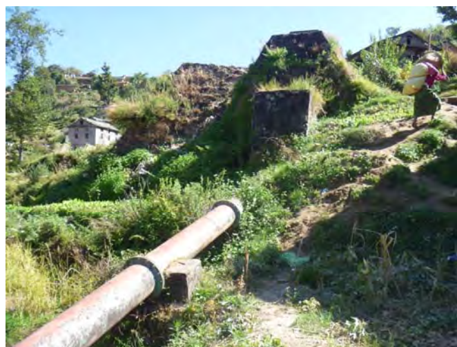
Figure 7-22 Head pond slope
