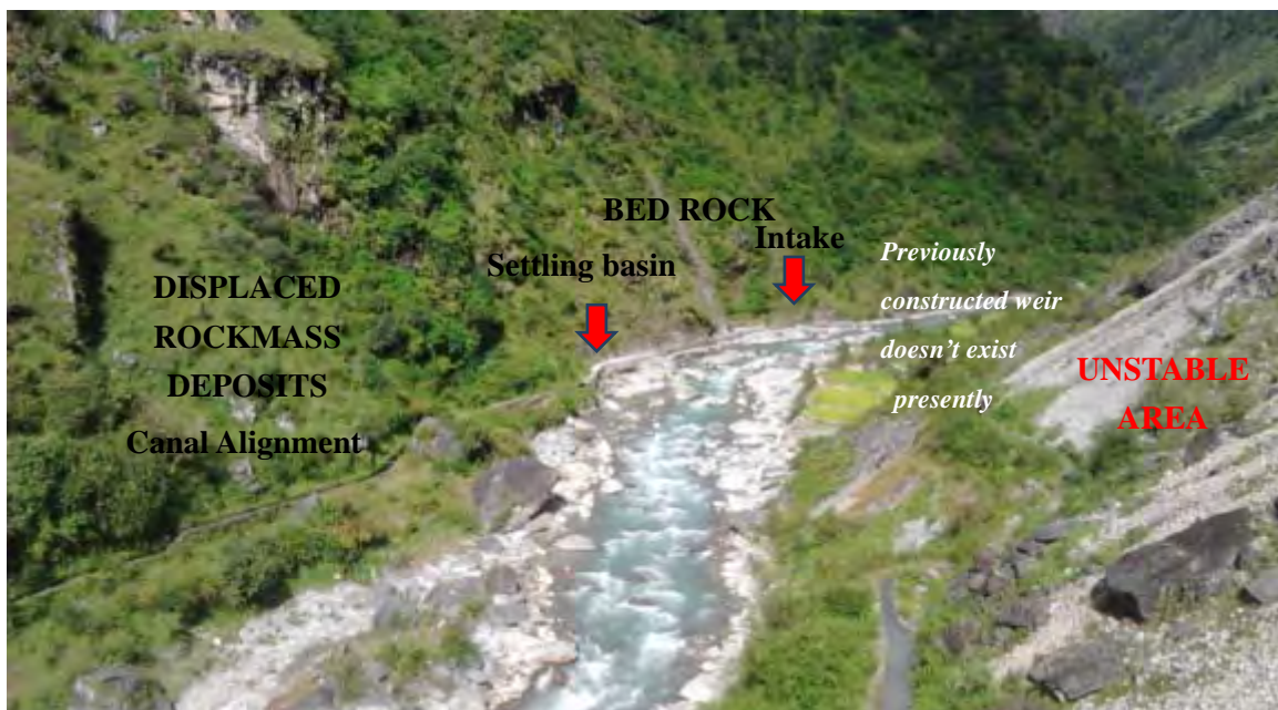
Figure 7-6 General Arrangement in Headworks Area
