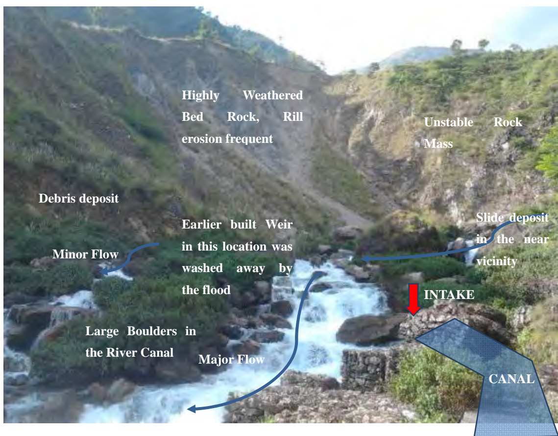
Figure 7-26 Engineering Geological Condition of the Headworks Area
