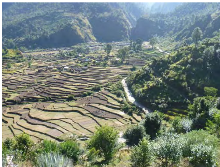
Figure 7-21 Headrace Channel slope
