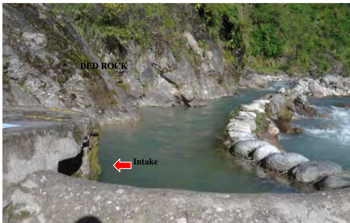
Figure 7-8 Bed Rock Exposed Near the Intake Area
