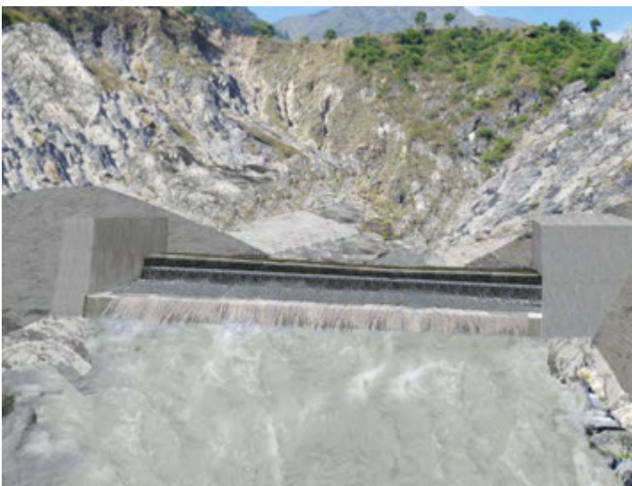
Syarpudaha Micro-hydropower Plant Intake
