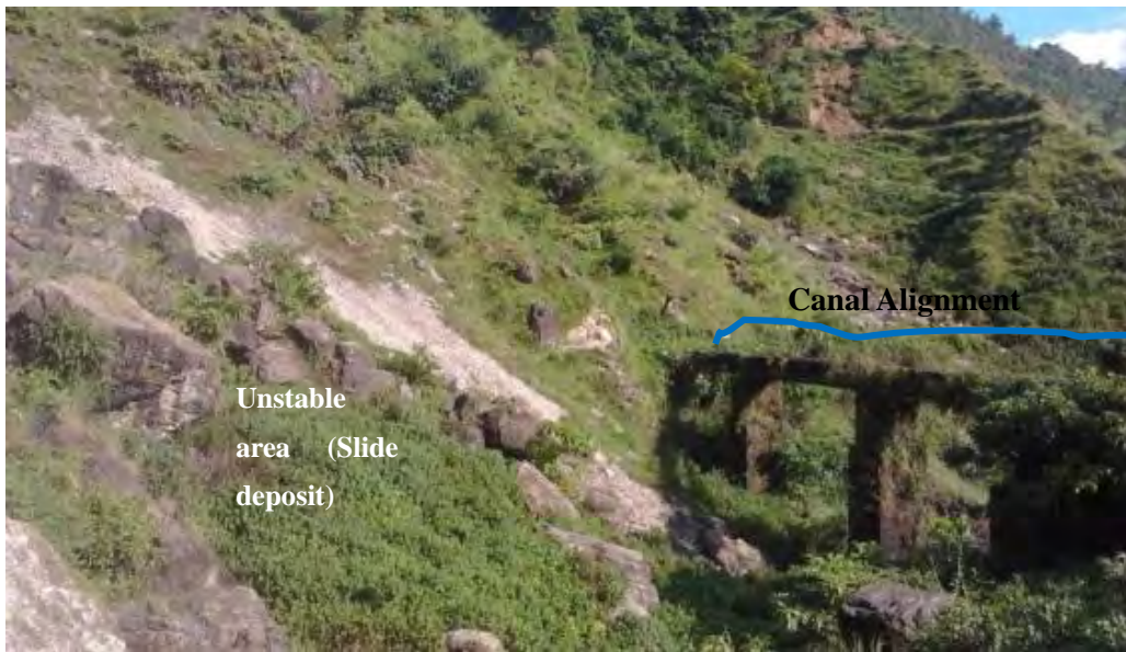
Figure 7-28 Support Pier between Chainage 0+000 and Chainage 0+100
