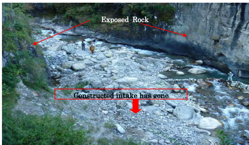
Figure 7-19 Intake photo (View from bridge)
