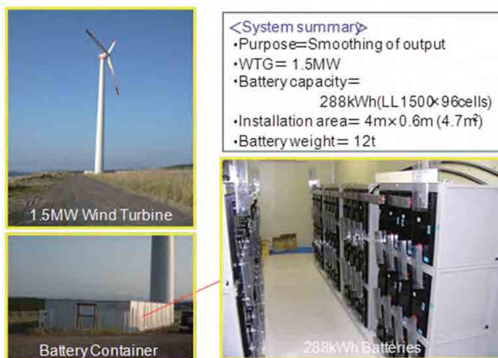
Figure 3-4-27 Demonstration wind park at Nishime (Akita, Japan)
