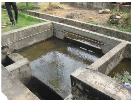
Photo 3.6 Chlorine Contact Tank
