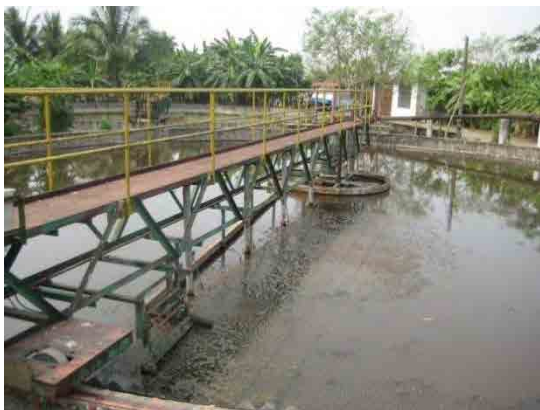
Photo 3.5 Final Sedimentation Tank
