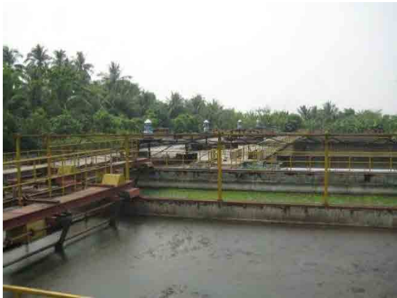
Photo 3.5 Final Sedimentation Tank
