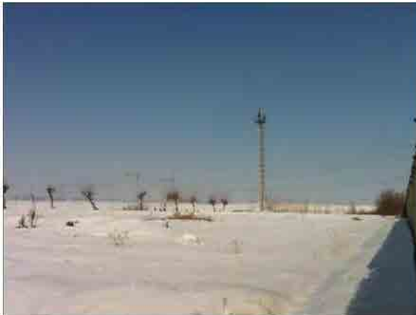
(a) New 220kV Switchgear Yard Space (1)
