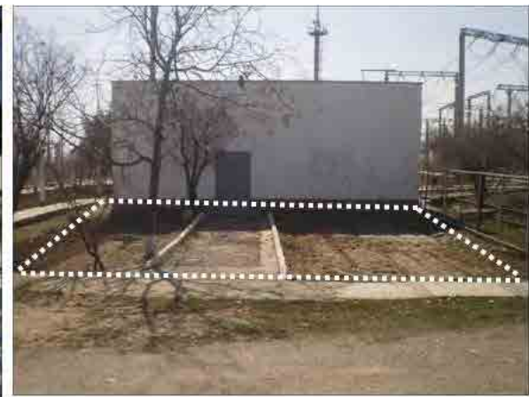
(f) New Control Building Space
