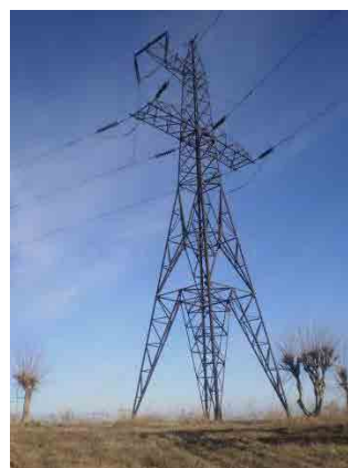
Figure 7.2.2-15 connection tower (Point K)
