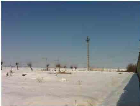
(a) New 220kV Switchgear Yard Space (1)
