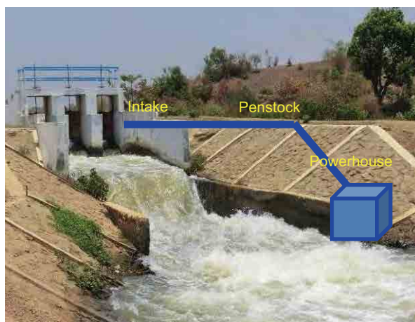
Figure 2.6.12 Conceptual Arrangement of Hydropower Plant at Bifurcation in Taung Nyo Irrigation System
