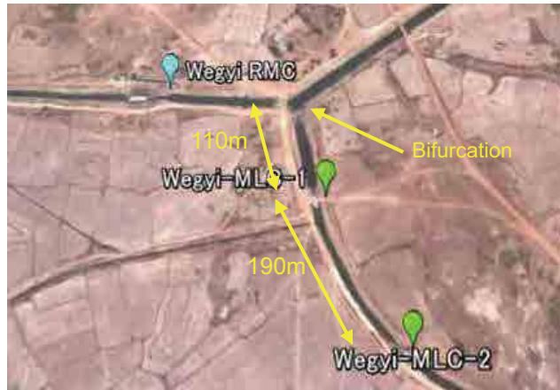
Figure 2.6.9 Locations of No.1 & No.2 Drop Structures in Left Main Canal of Wegyi Irrigation System
