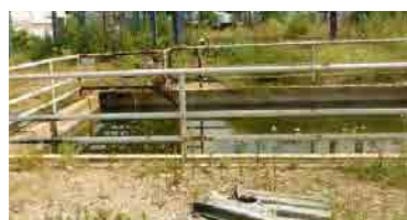
Sedimentation tank for discharged water which comes from the electrolysis plant
