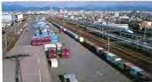
Freight Station (Japan, Kyoto Freight Station)
