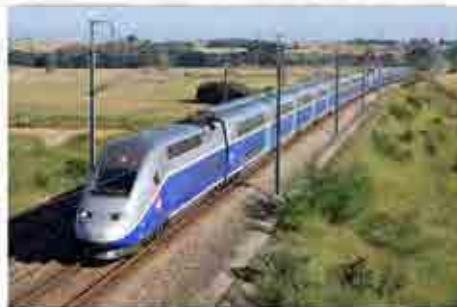
Earthworks, TGV Sub-Est
