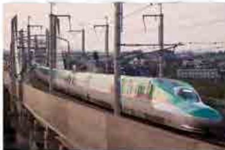
Extradosed Bridge, Tohoku Shinkansen
