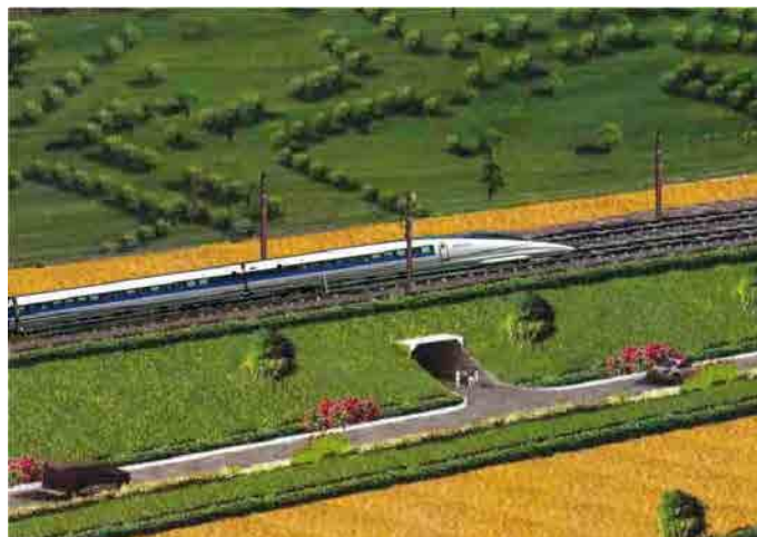
Figure 10.1 Image of Embankment with a Box Culvert
