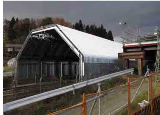
Tunnel Entrance Hood
