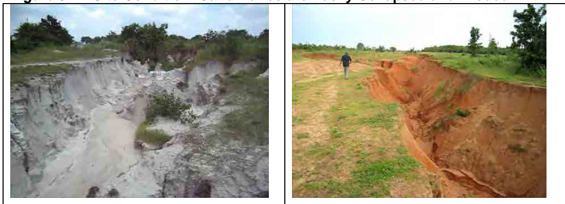
Figure 3D.4 Site Condition: Sand Dunes are Easily Collapsed and Eroded
