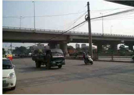
Road Over Bridge (Ring Road No.3) (View toward Ngoc Hoi)
