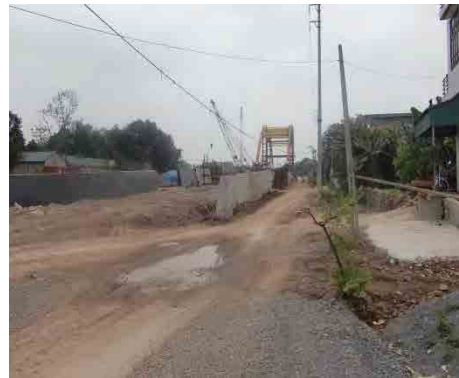
(Development Work Started)
