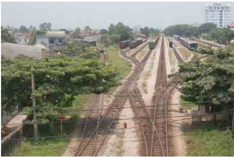
Overall View of Vinh Station (from road flyover)
