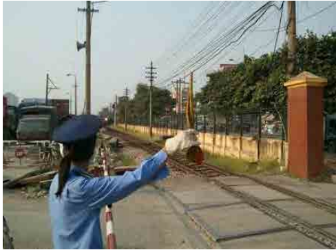
Level Crossing (KM 5+490) (View toward Hanoi)
