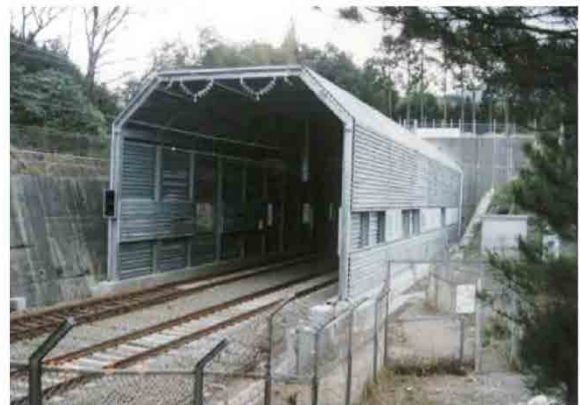
Figure 5B.3 Two Cases of Buffer Tunnel for Shinkansen
