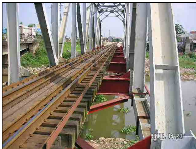
Figure 5.3.25 Bridge Sleeper Track between Hanoi and Ninh Binh
