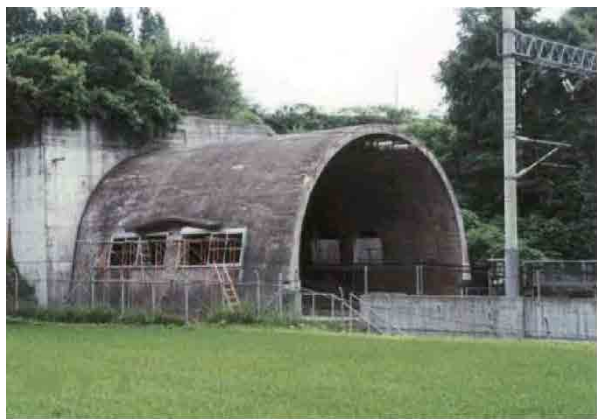
Figure 5B.3 Two Cases of Buffer Tunnel for Shinkansen
