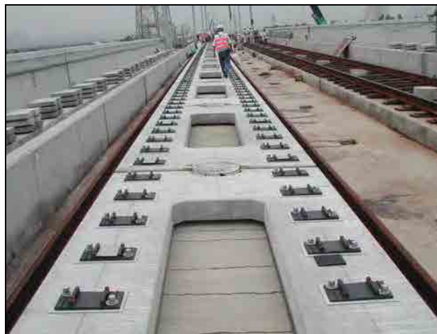
Figure 5.3.23 Viaduct Section with Frame Type Slab Track in Taiwan High Speed Railway
