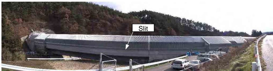
Figure 5B.4 A Slit Shelter Installed for Shinkansen
