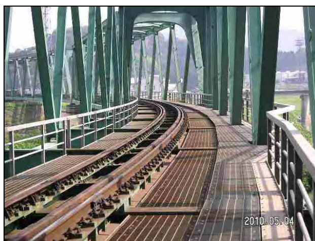
Figure 5.3.25 Bridge Sleeper Track between Hanoi and Ninh Binh
