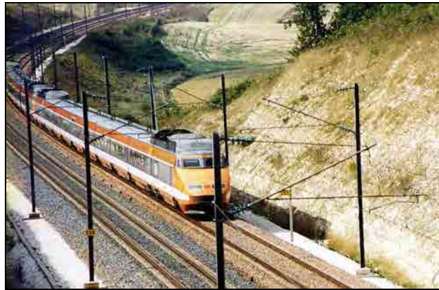
Figure 5.2.3 Earthwork Section and Ballast Track in TGV Sud-Est Line
