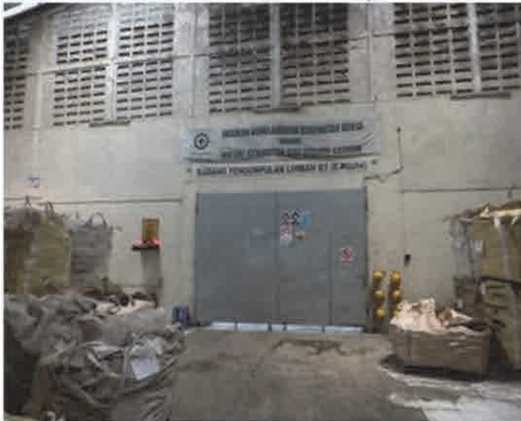
Inside of collection facility (1)
