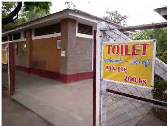
Public toilet from outside
