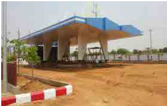
Gas station is constructed besides of bus terminal
