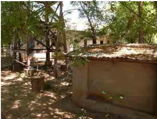
Well and elevated tank
