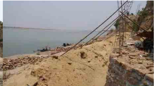
Bank protection work on the Irrawaddy River 2
