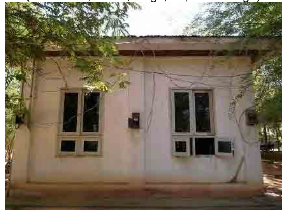
Electric meter and electric wire
