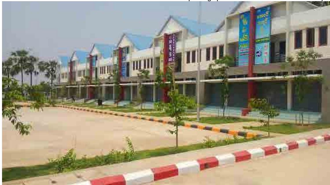
New Bus terminal almost completed
