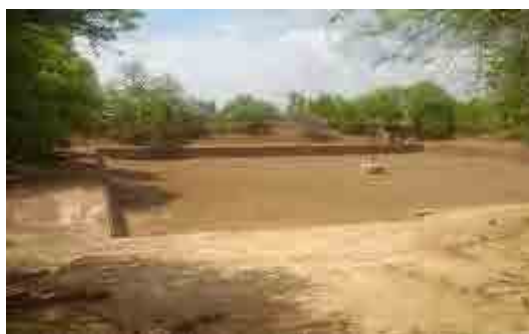
Water reservoir built in the 13th century at Min-nan-thu Village (37mX37 mX4mH). Dried-up during dry season, so only being used in rainy season
