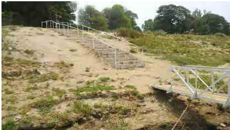
Simple stairway and pier, which are rebuilt every year after the submergences.
