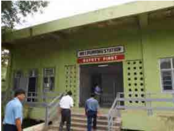
Pump station No.1 After pumping up from the river, it will be pumped up to pump station No2.
