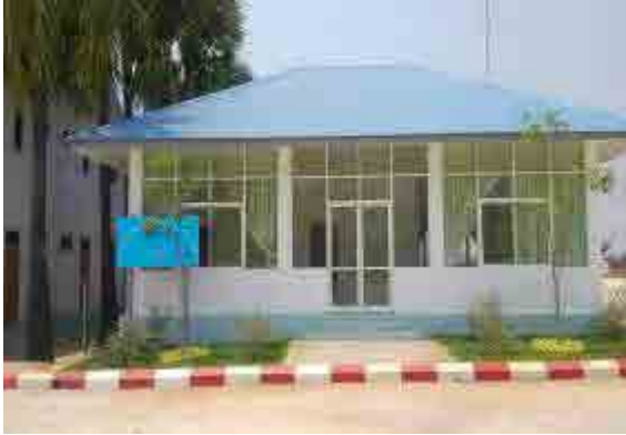
Administrative office in bus terminal
