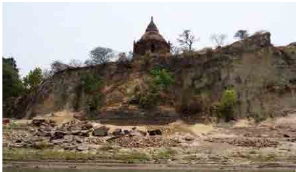
Bank protection work on the Irrawaddy River 1
