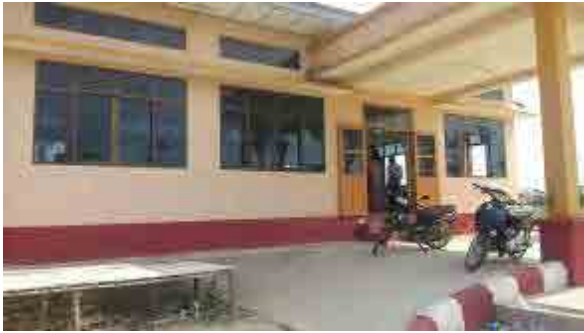
Substation (2) in Nyaung-U Town constructed in 2013
