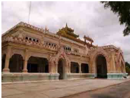
Nyaung-U Railway Station (Established in 1996)
