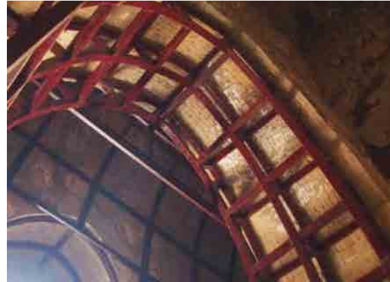
Reinforcement for vault arch
