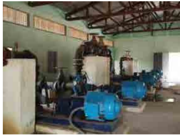
Pump station No.2 After sending water to settlement basin, water will be delivered to towns and villages.
