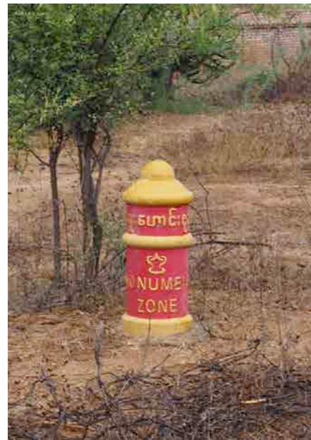
Post installed in the zoning boundary
