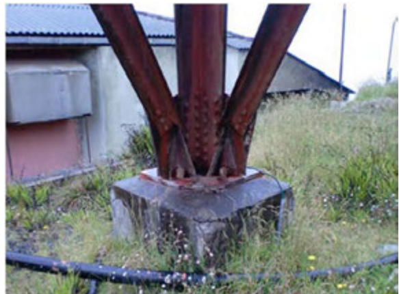
Basement of tower at Pidurutalagala station
