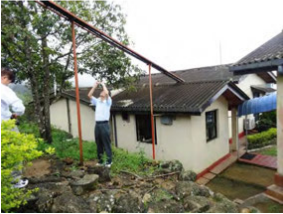
Feeder checking by JICA Study team at Karaghatenna transmitting station
