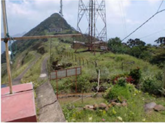
Suriyakanda transmitting station of ITN
