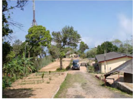
Yatiantota transmitting station
