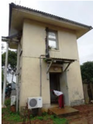
Primrose Transmitting station of SLRC
