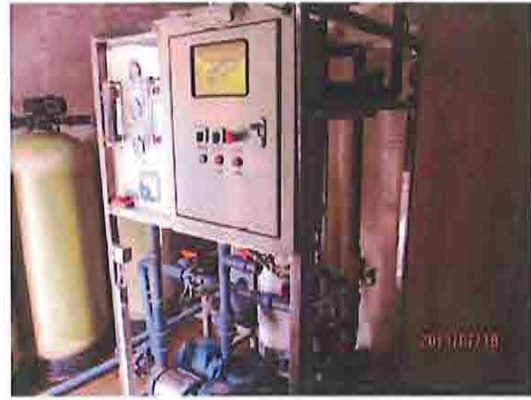
Center : Control Panel Left : Adsorption Tank, Right : Effluent Storage Tank
