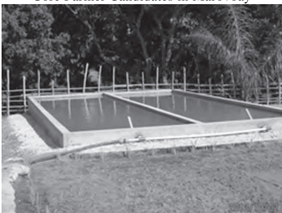
Concrete Tanks of a Core Farmer in Mahajanga II
