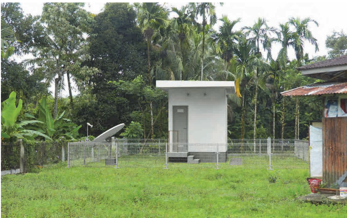
Image of Completion (with fence) No.70 BONJOL Seismic Station
