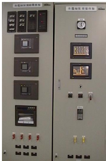
Figure4-29 Design of Integrated Control Panel
