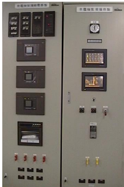
Figure 4-36 Design of Integrated Control Panel
