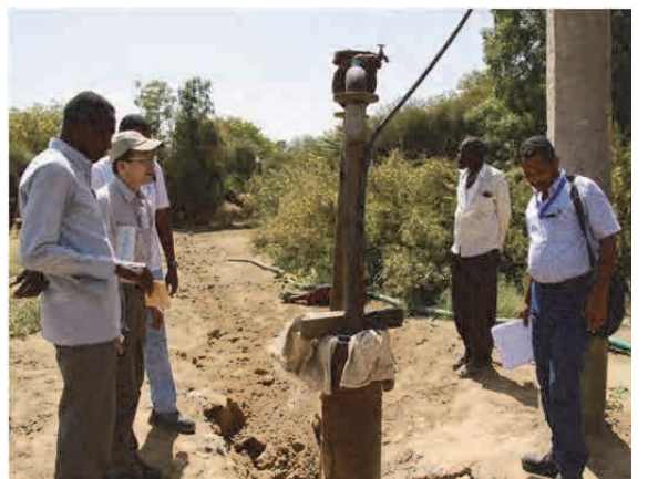
Borehole rehabilitated by SWC during SMAP phase-1. In phase-1, total 14 water facilities were rehabilitated in West Darfur.
