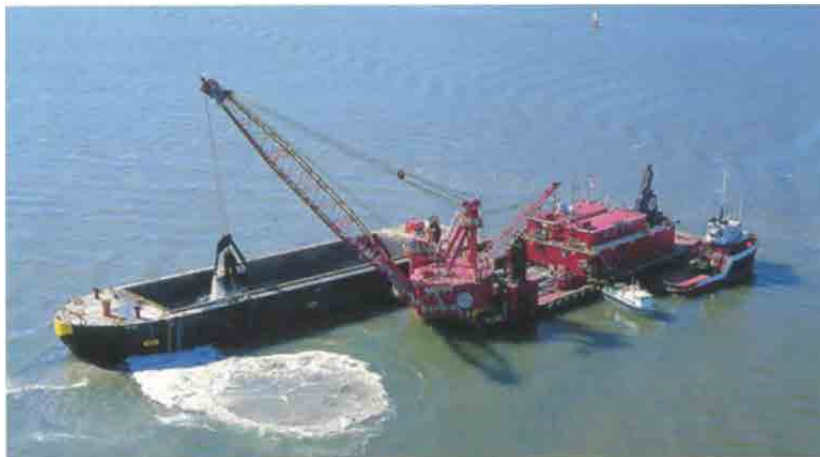
Photo 5.4 Grab Dredger (pontoon type)
