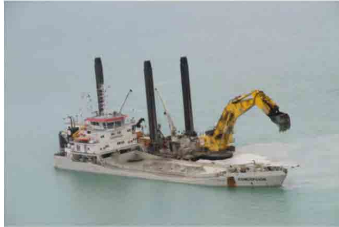
Photo 5.5 Backhoe Dredger (Source: “Mimar Sinan” Jan De Nul Group)
