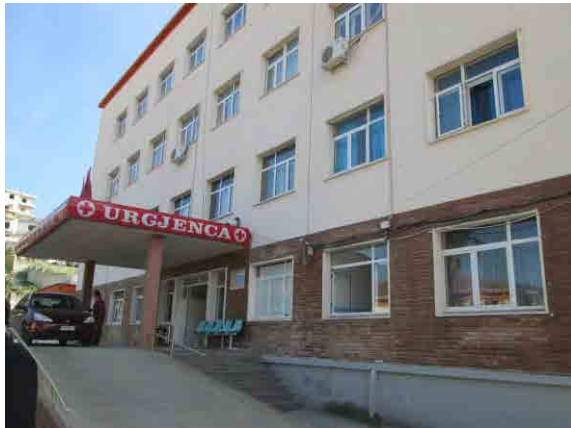
7. Vlore Regional Hospital
