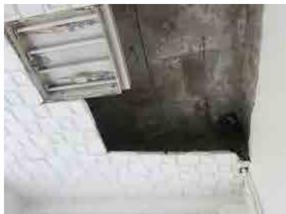
17. UCCK Facilities under renovation
