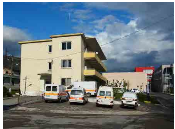
6. Elbasan Regional Hospital Laboratory and emergency wards
