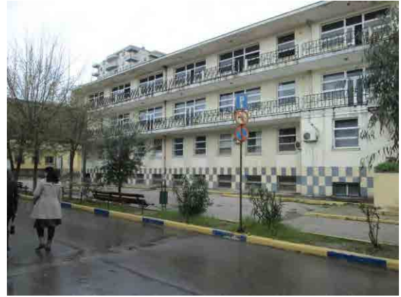
2. Durrës Regional Hospital An pediatric ward of under renovation
