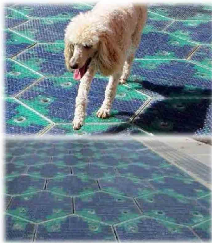
Figure 3.53 Road Pavement with Solar Panels
