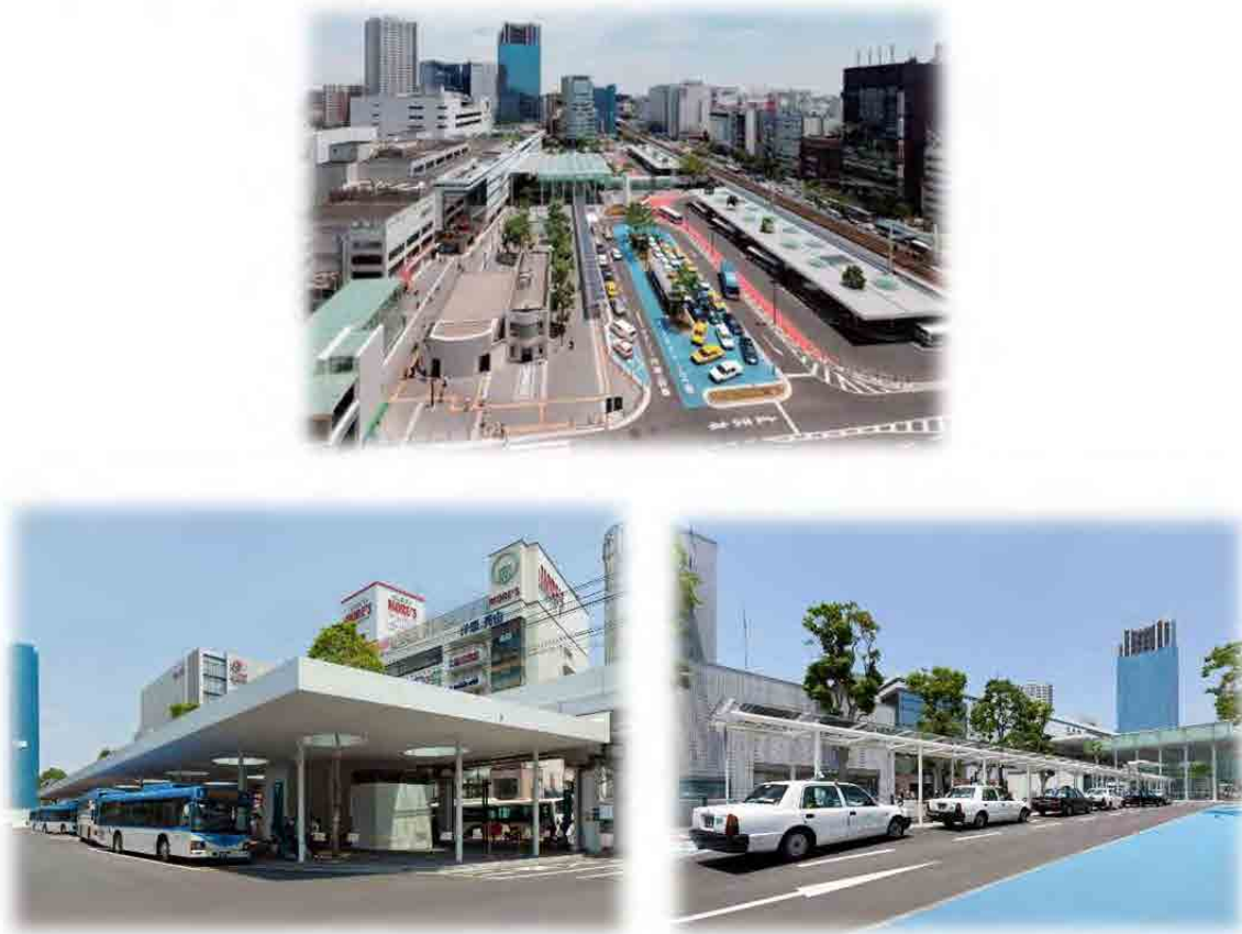
Figure 3.51 Separated Locations of Taxi and Bus Stops (Kawasaki City in Kanagawa Pref.)
