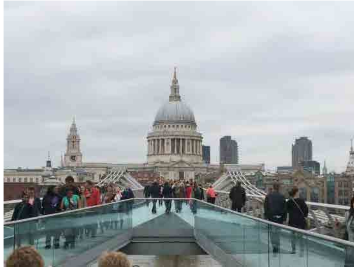
Figure 3.67 Example of Pedestrian Bridge (London)
