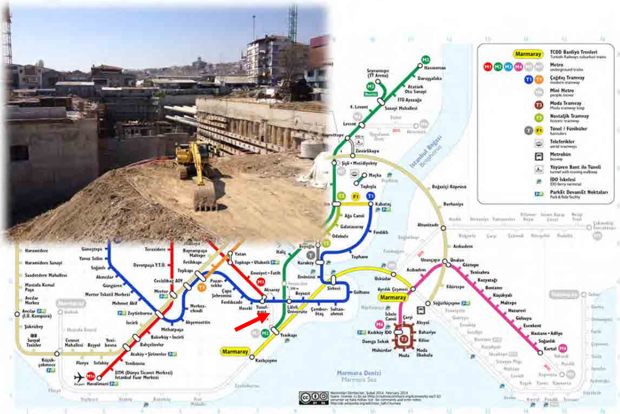
Figure 3.5 Construction of LRT Yenikapi Station
