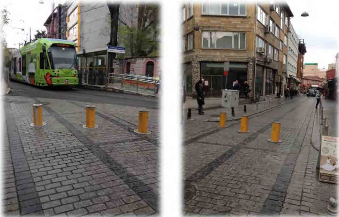
Figure 3.31 Vehicle Stopping Barrier in other area
