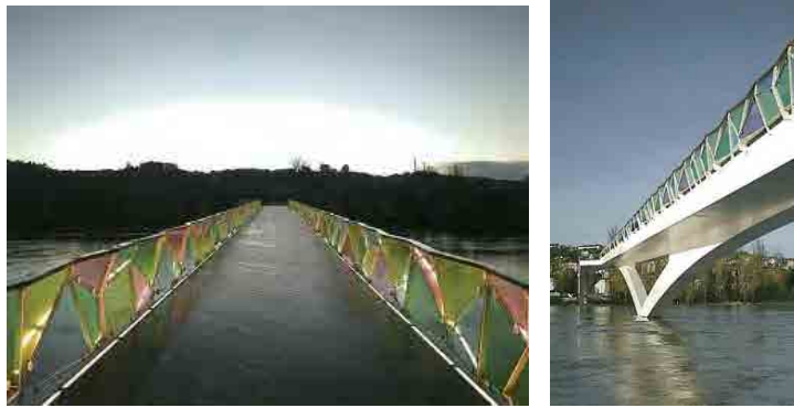
Figure 3.68 Example of Pedestrian Bridge (PORTUGAL, Coimbra city)
