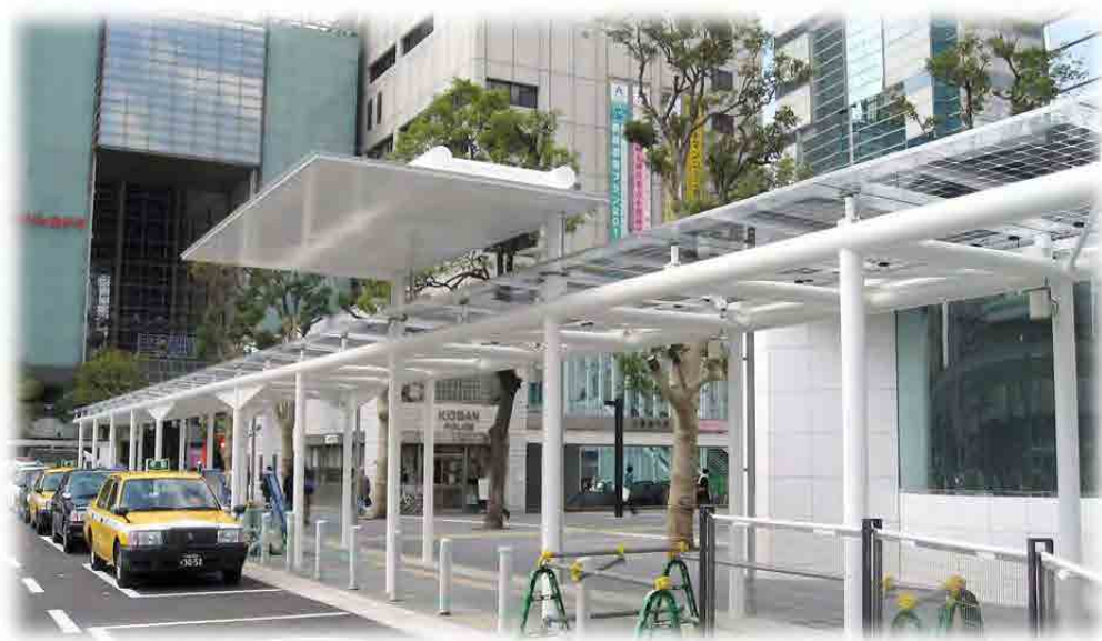
Figure 3.52 Taxi Stops with Roofs Solar Panel
