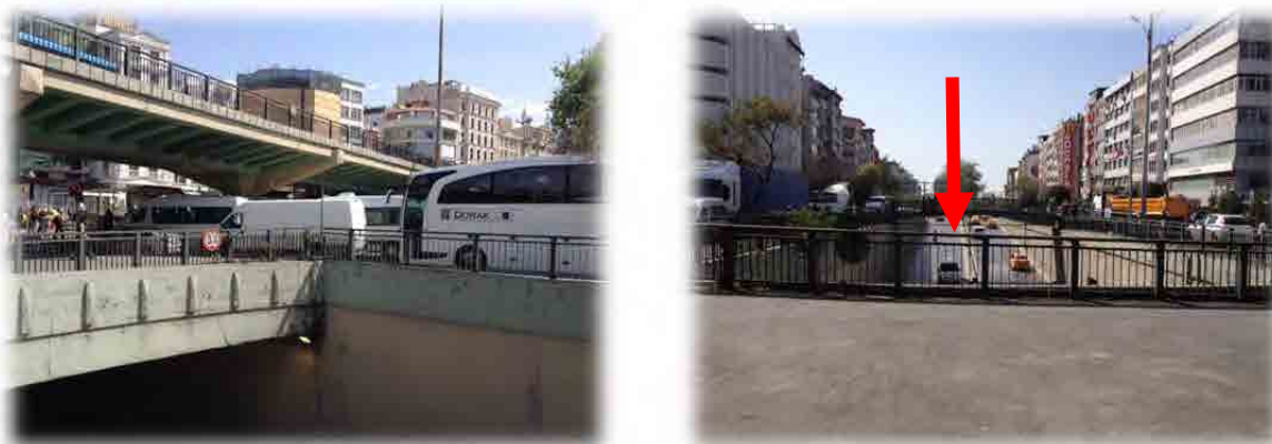
Figure 3.9 Under Pass and Pedestrian Bridge around the Aksaray Station of Tramway
