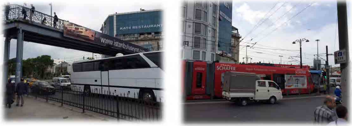
Figure 3.22 Pedestrian Bridge and Tramway around Sirkeci Station Area
